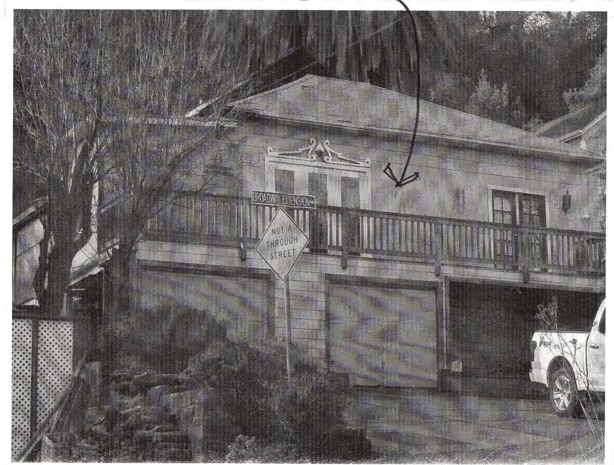
PHOTO OF EXISTING STRUCTURE
