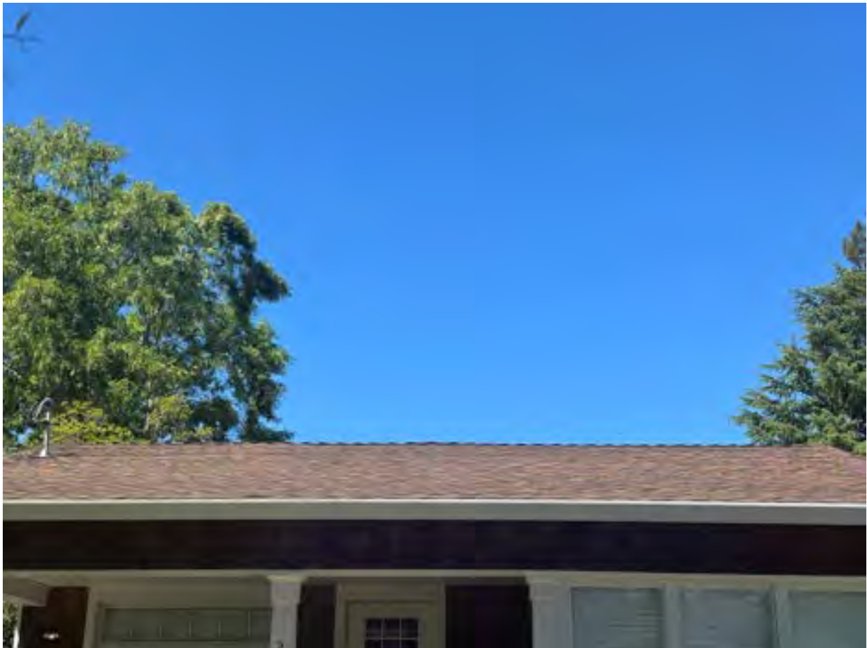
Figure 8. Roof Material: Composite Shingle
