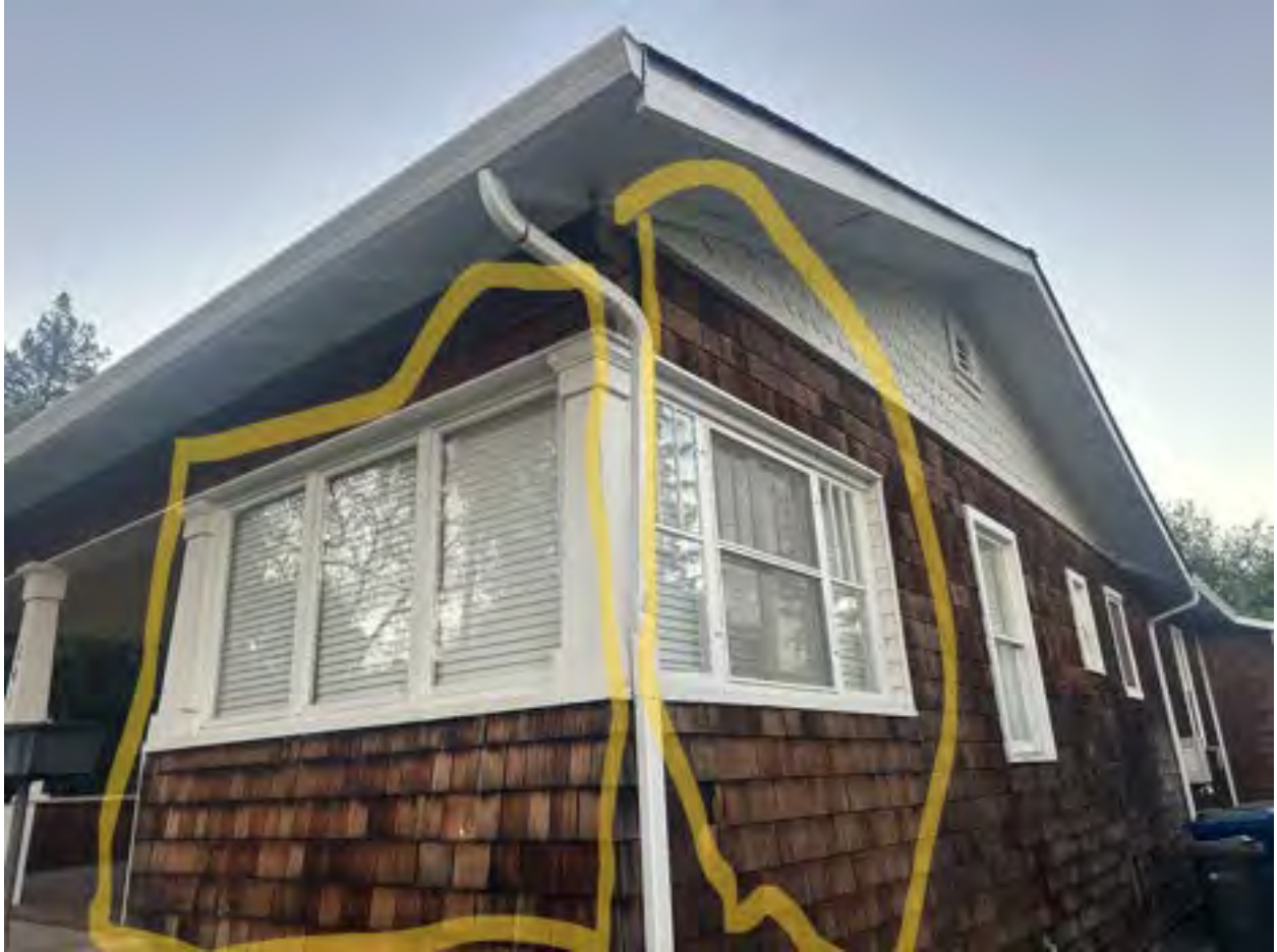
Front Façade + North Side post-1956 Constructions (Marked Areas)
