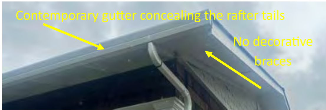
Figure 4. Covered Roof Rafters post-1990
