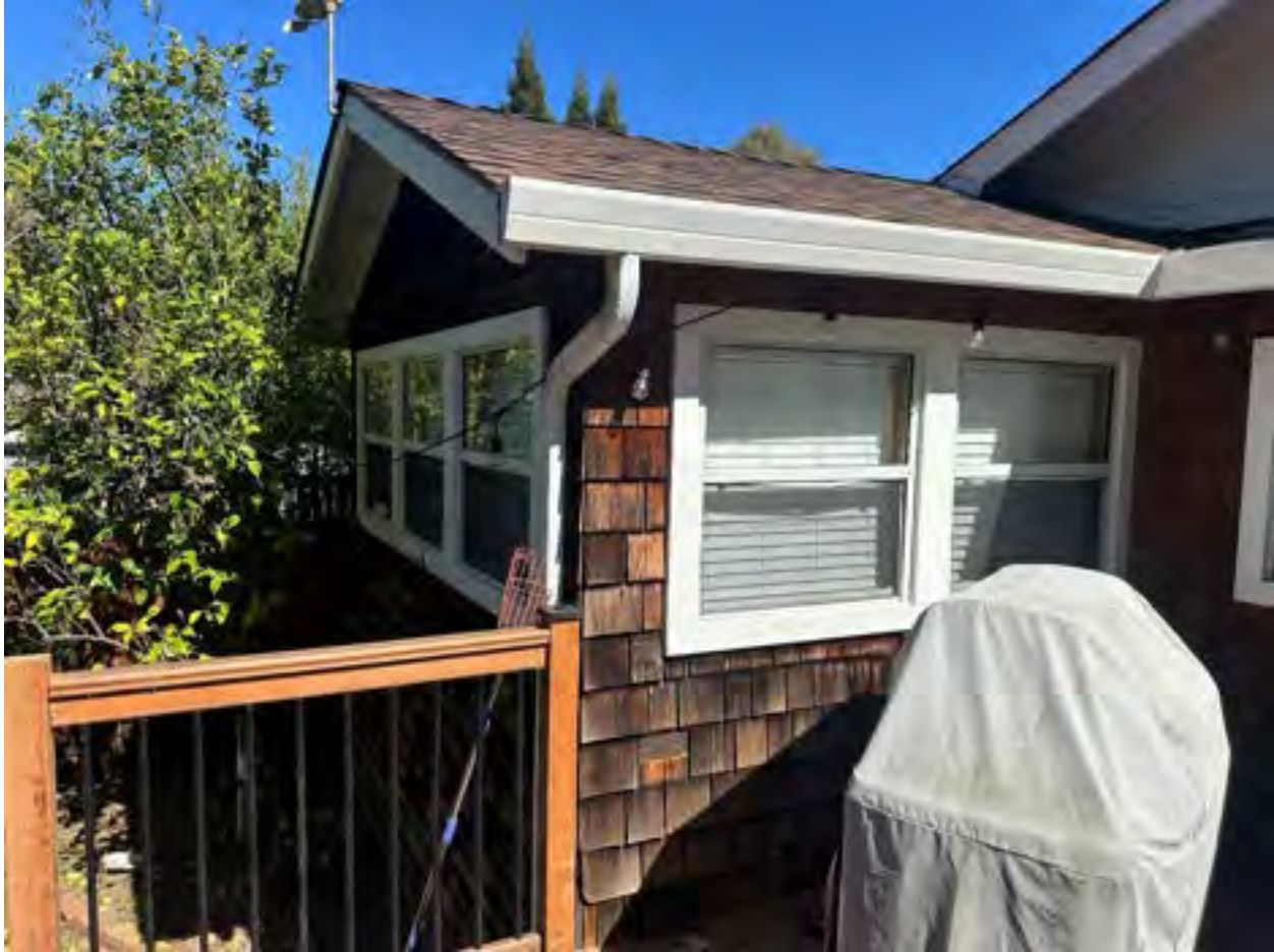
Rear Side post-1956 Constructions
