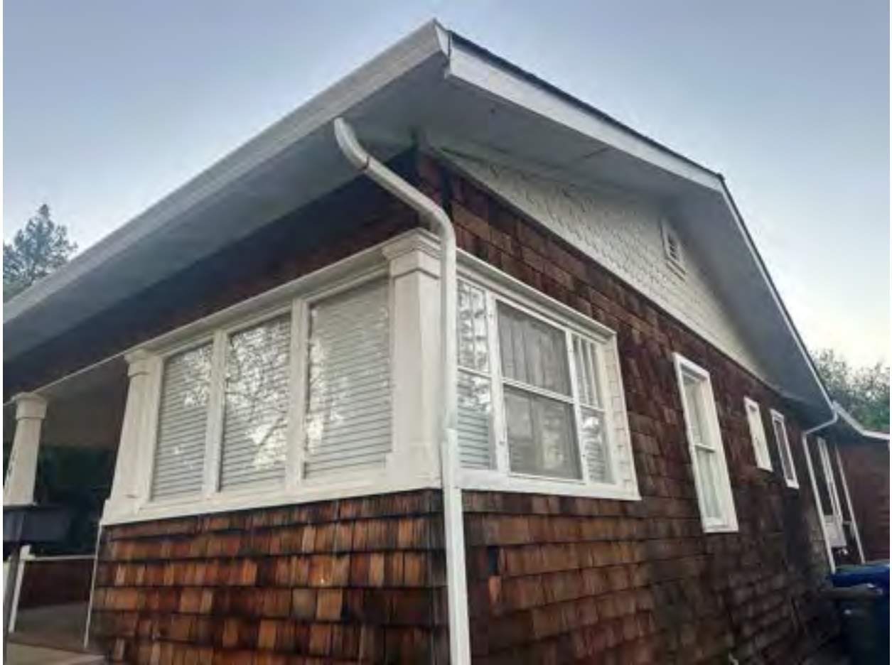
Front Façade + North Side post-1956 Constructions
