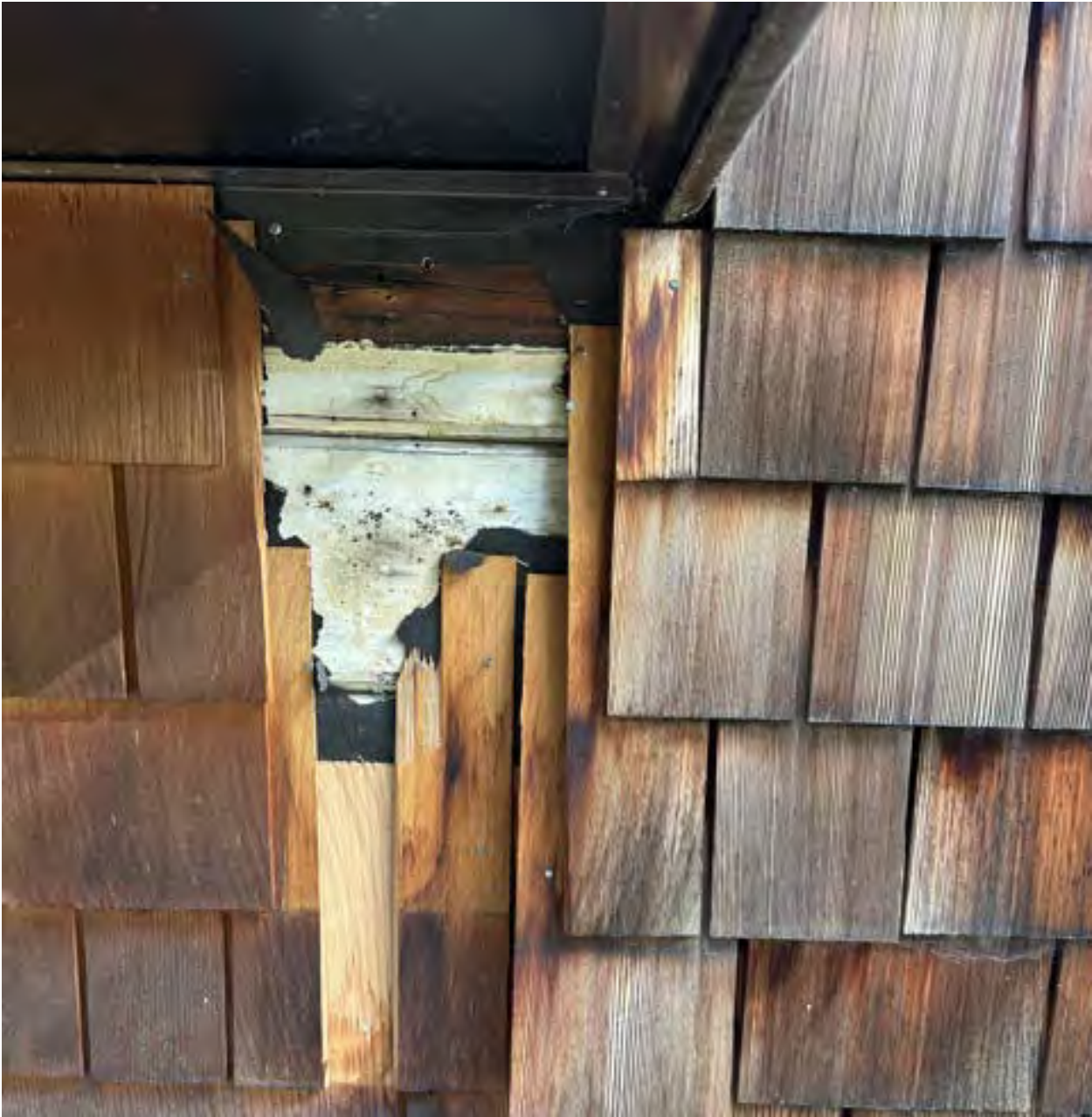
#6: South Side – Middle (original siding):
