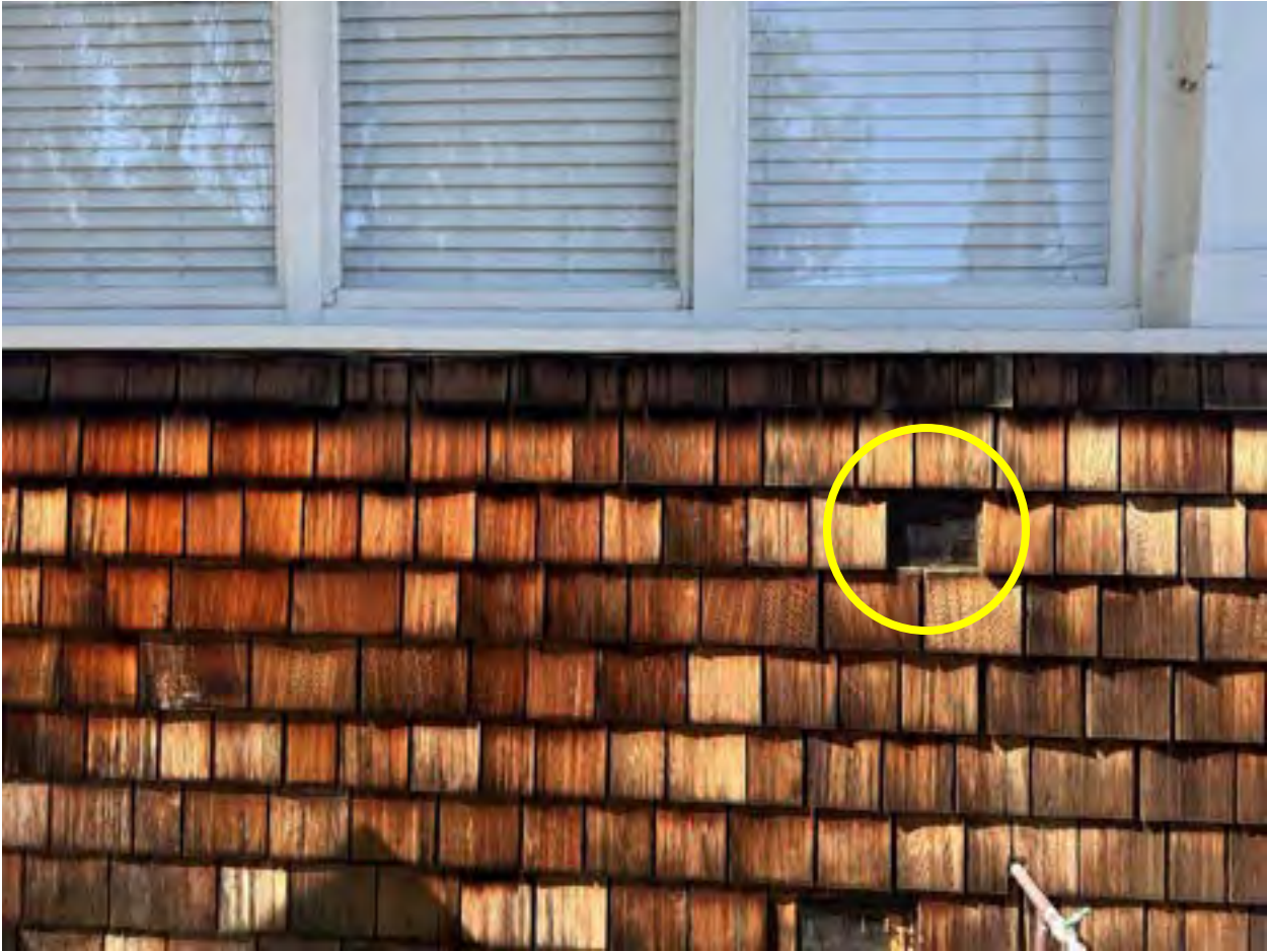
#1: Front Façade – Right:
