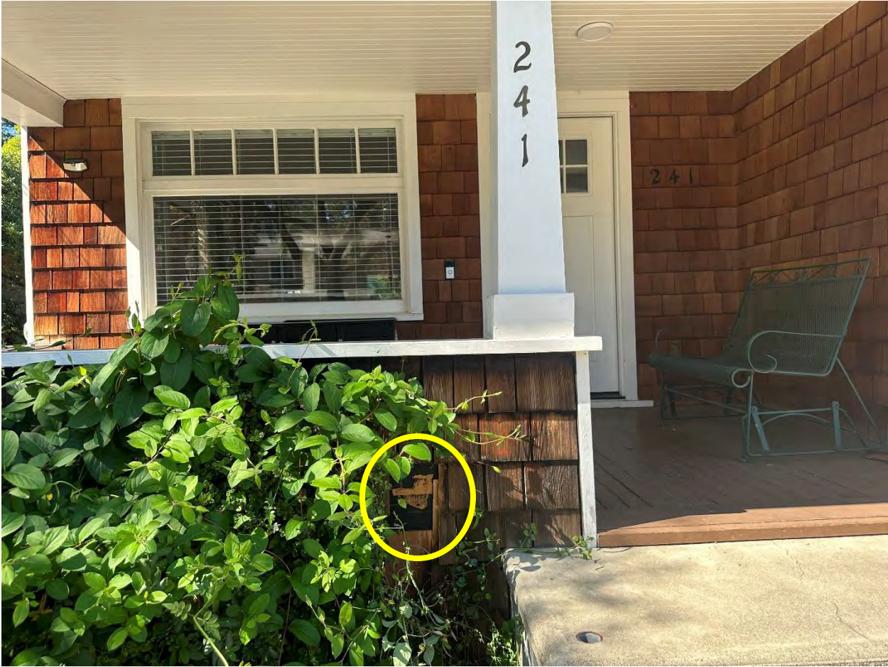
#2: Front Façade – Middle-Left:
