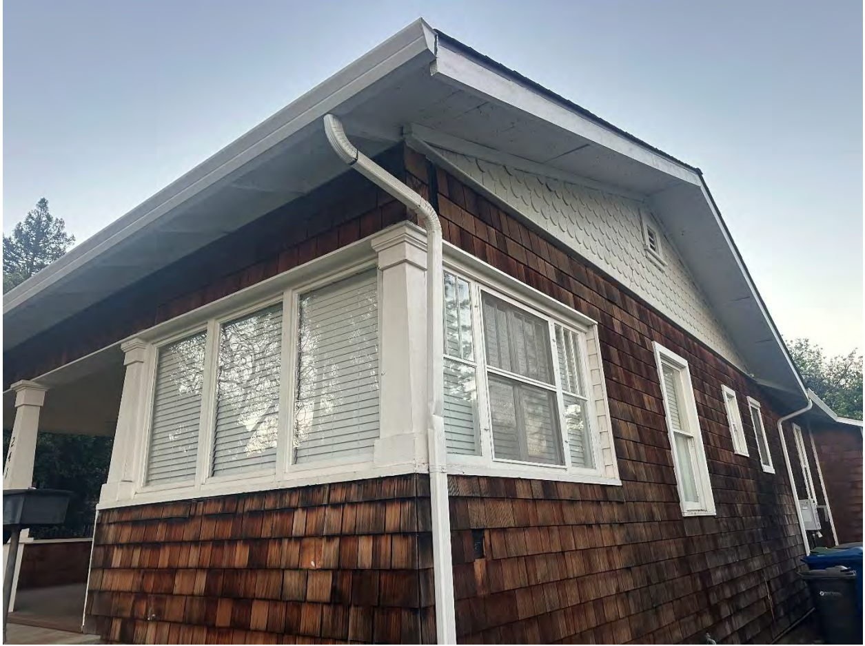
Front Façade + North Side post-1956 Constructions
