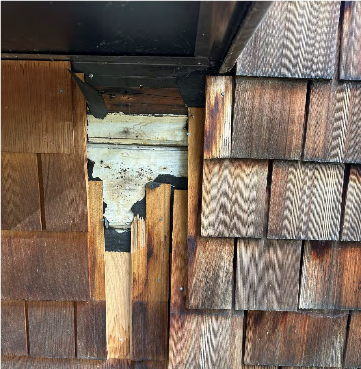
#6: South Side – Middle (original siding):
