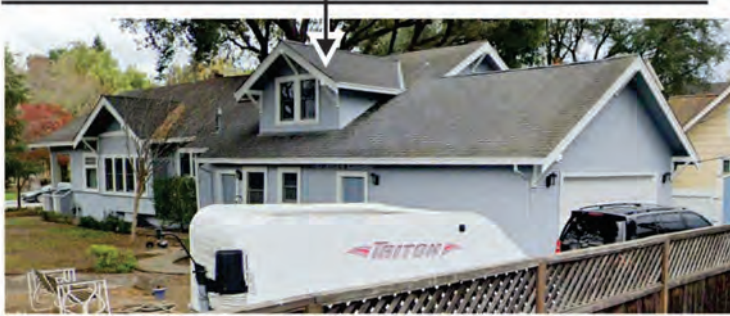
Second floor addition was treated as a dormer with a ridge line lower than the main roof which is consistent with the original architectural style of the house
