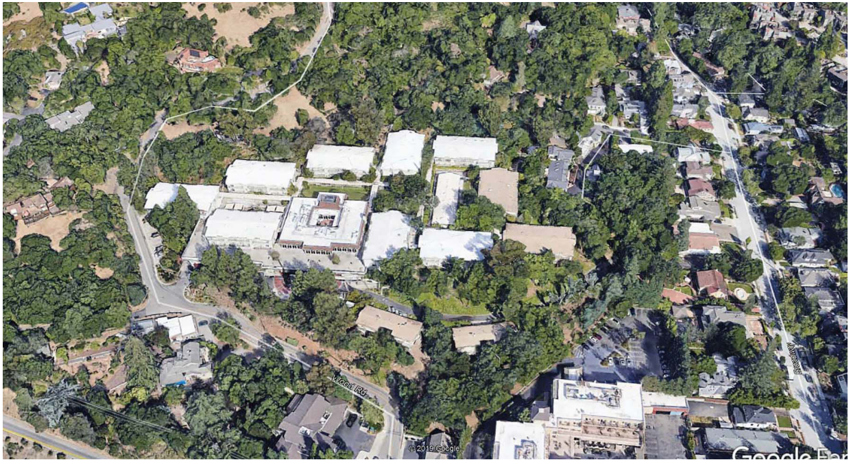
Aerial view of site from the east
