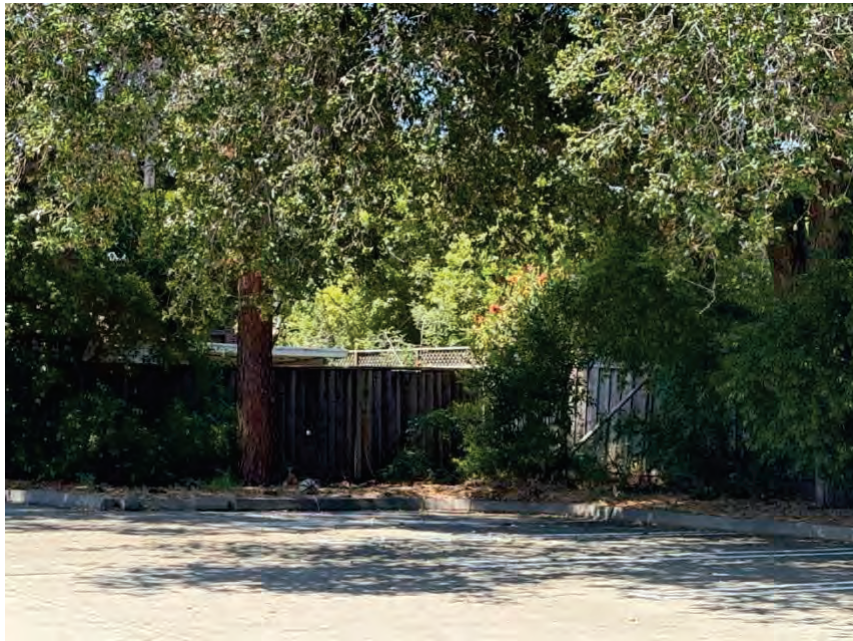
D-E – Farley west fence
