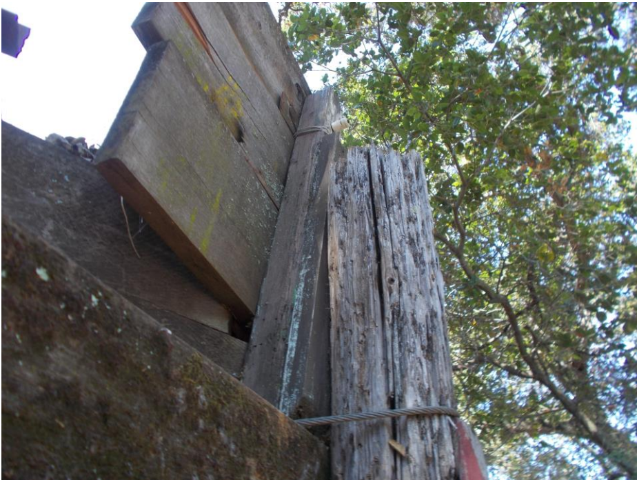
Photo 2 – Top of wall extended 3 boards (3 feet) to support raised parking pad.
