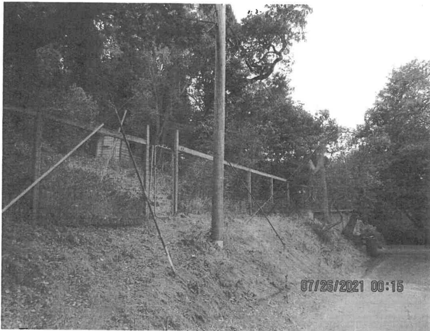
45 Reservoir Rd, Story poles and unpermitted tree removal
