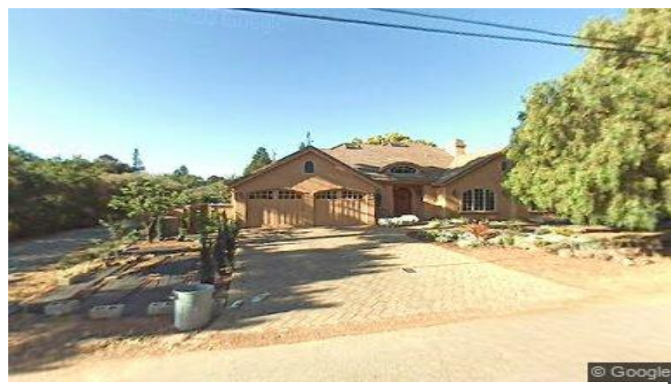
446 San Luis Ave, Los Altos HOUSE STYLE: MODERN NUMBER OF STORIES: 2 EXT. MATERIALS: STUCCO ROOF STYLE: GABLE ROOF MATERIALS: COMP SHINGLE
