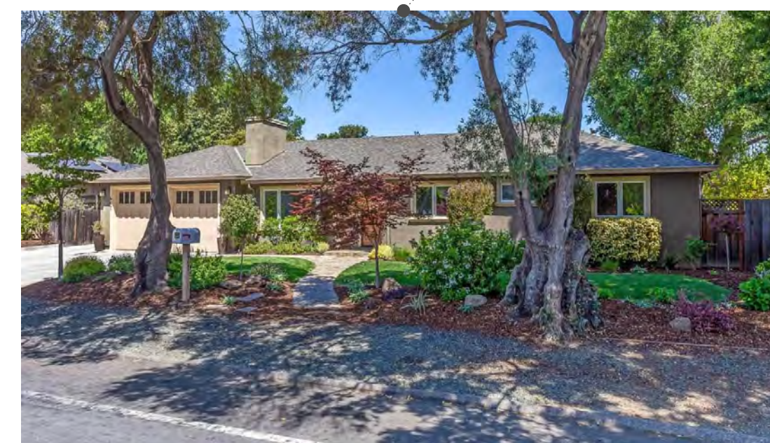
467 CUESTA DRIVE HOUSE STYLE: TRANSITIONAL NUMBER OF STORIES: 1 EXT. MATERIALS: STUCCO ROOF STYLE: HIP ROOF MATERIALS: COMP SHINGLE
