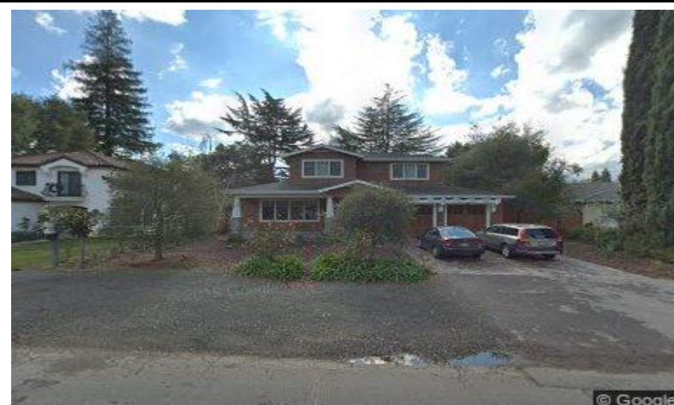
452 Paco Dr, Los Altos, CA HOUSE STYLE: TRANSITIONAL NUMBER OF STORIES: 2 EXT. MATERIALS: WOOD ROOF STYLE: HIP/GABLE ROOF MATERIALS: METAL
