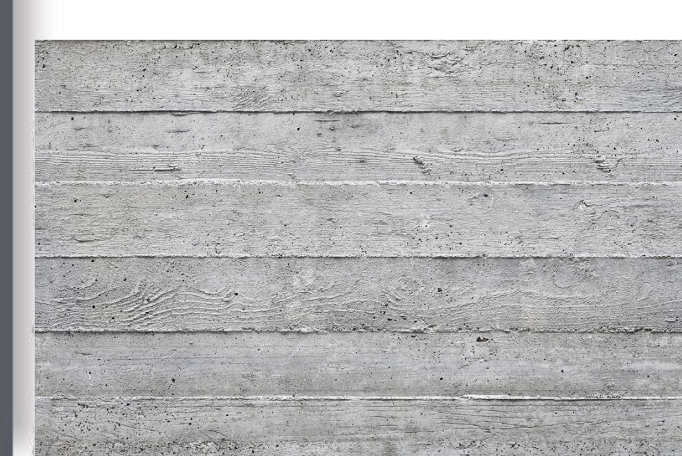
BOARD-FORM CONCRETE LANDSCAPE WALLS
