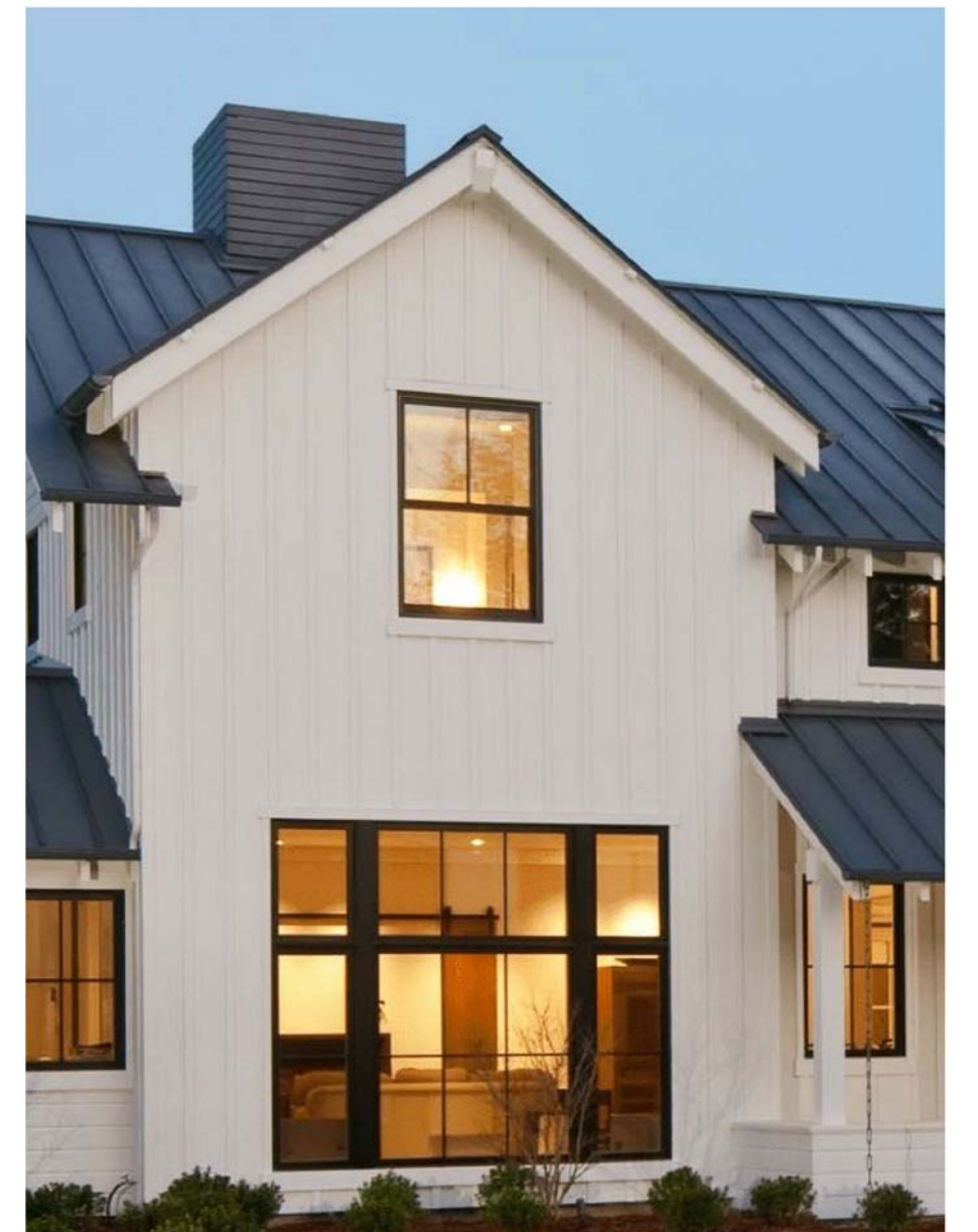
FIBERGLASS WINDOW FRAME (DARK COLOR) WITH WOOD TRIM (LIGHT COLOR) MANUF.: MARVIN OR SIMILAR
