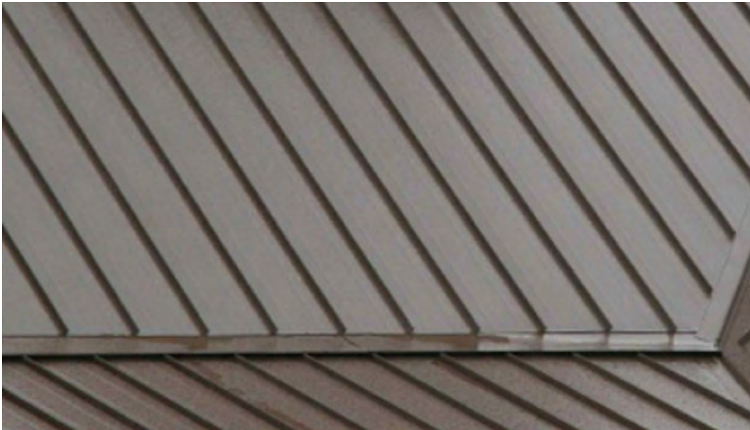
Roof: STANDING SEAM METAL ROOF Dark bronze
