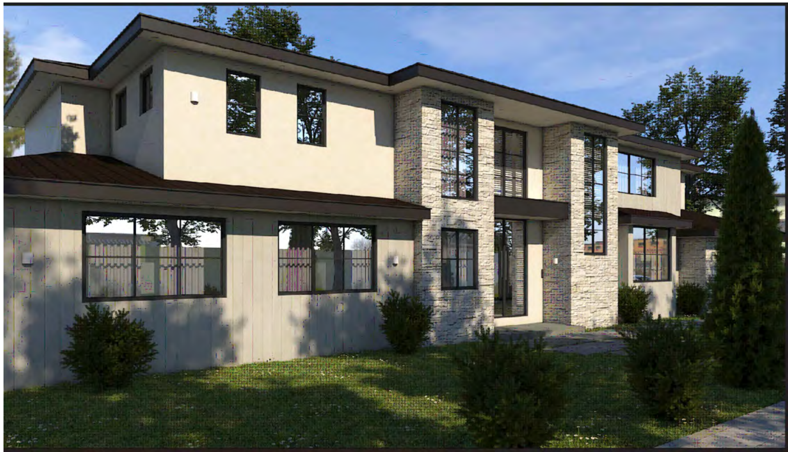
3 FRONT SOUTH WEST FACADE
