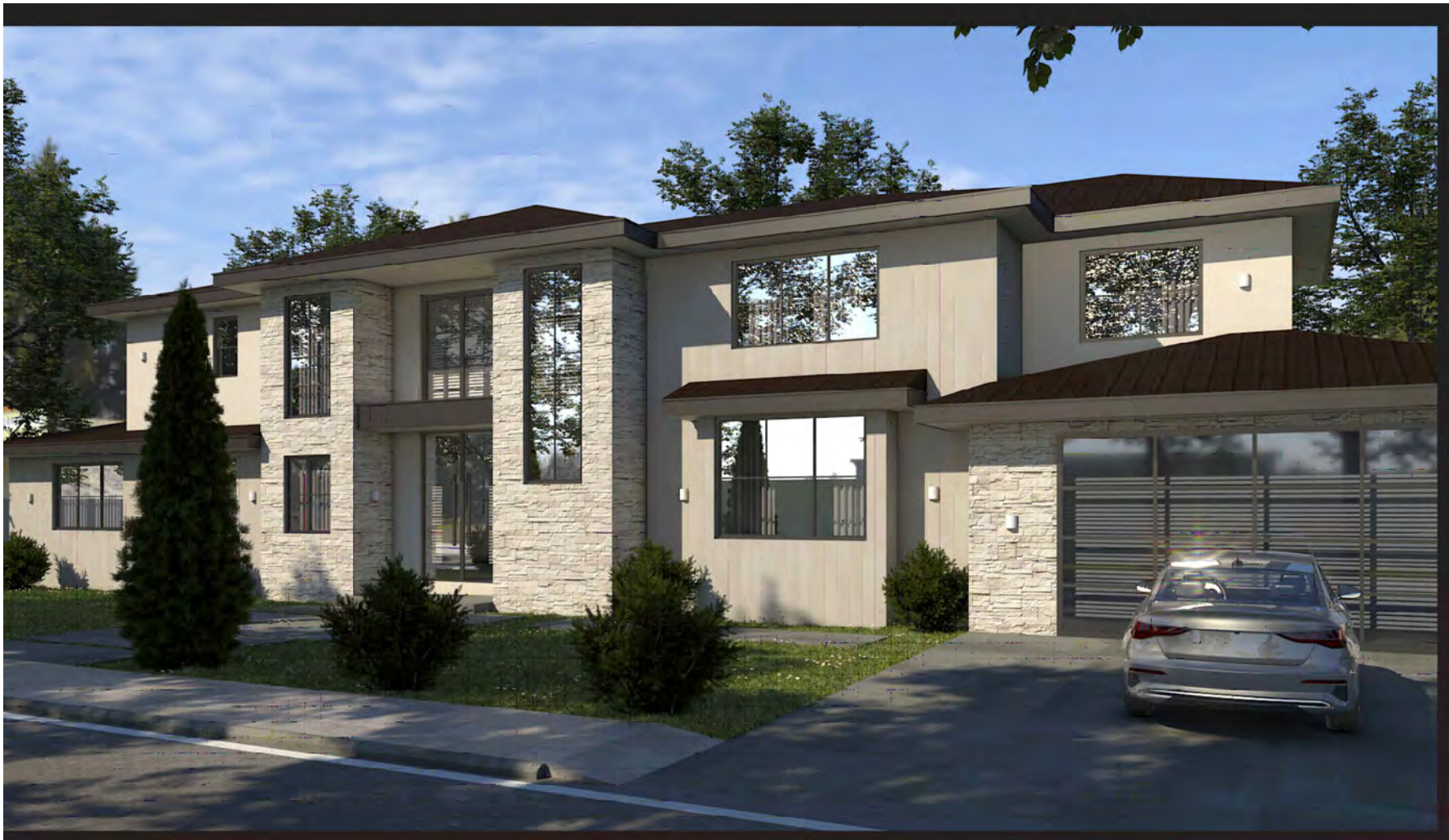
2 FRONT SOUTH EAST FACADE
