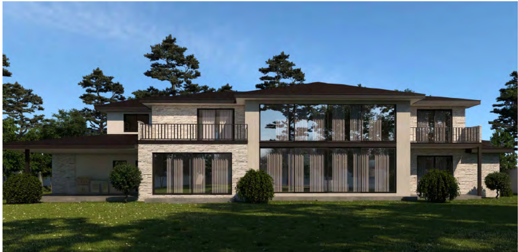
4 REAR NORTH FACADE
