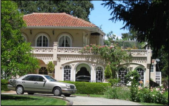
Figure 1: Existing Historic House
