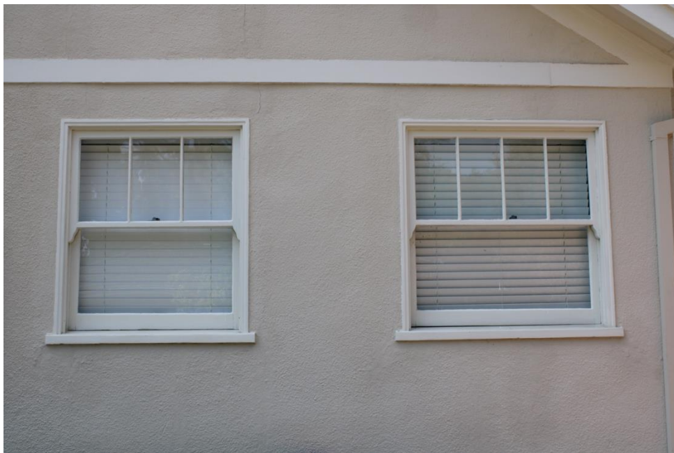
Figure 33. Three-over-one windows with horned stiles (aka lugs) on the east elevation, facing west.
