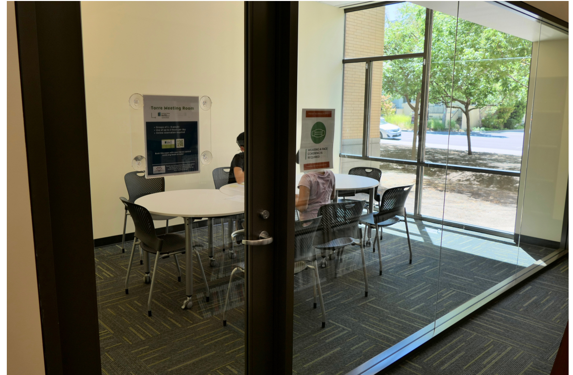
Glass panels connected with caulking
