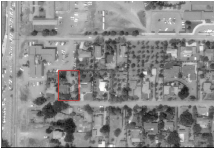
Figure 27. 1968 aerial photograph of the Property with increased residential development around it (courtesy of the University of Santa Barbara Library).
