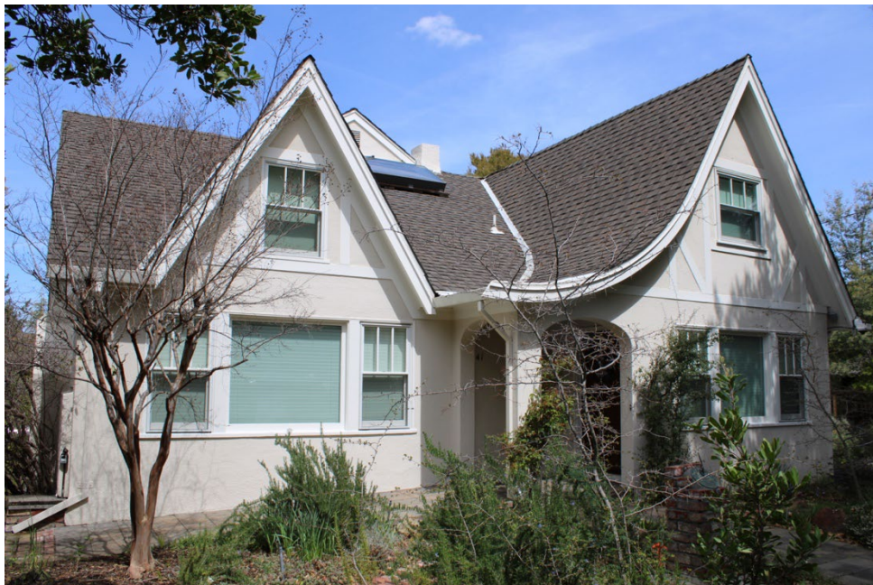
Figure 2. South elevation, facing northeast.
