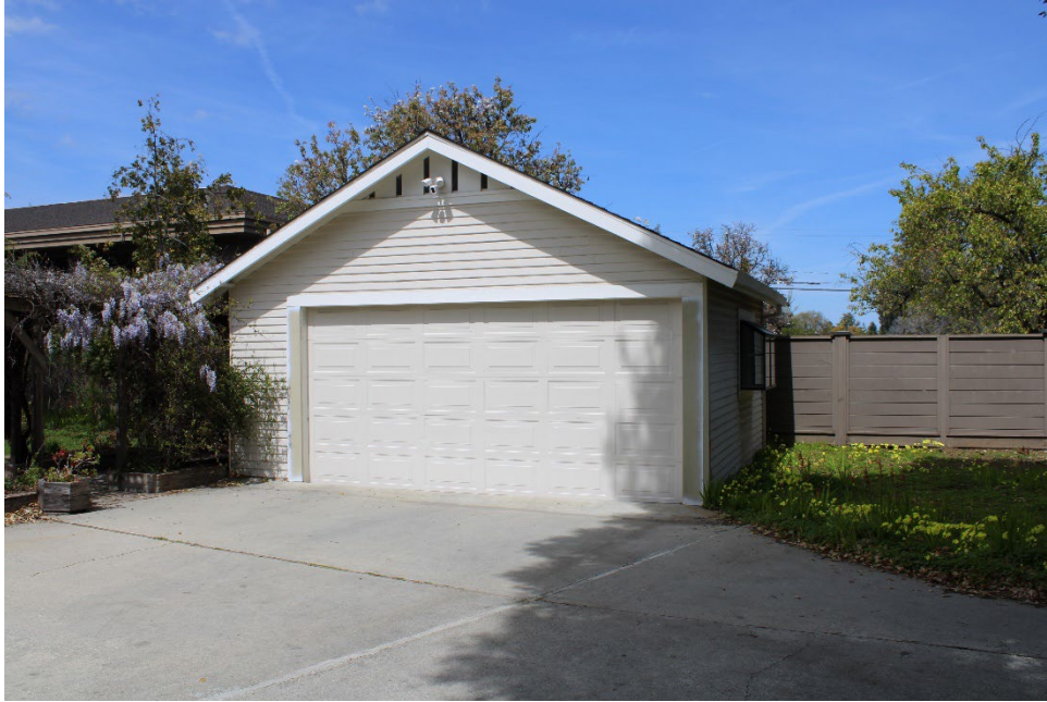
Figure 11. South elevation of detached garage, facing north.
