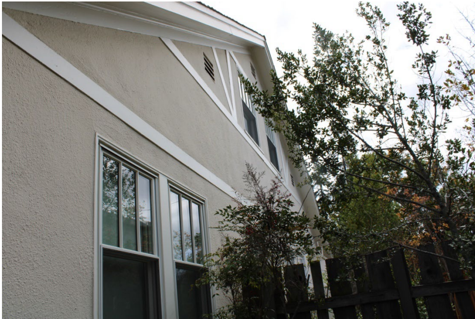
Figure 9. West elevation, facing southeast.
