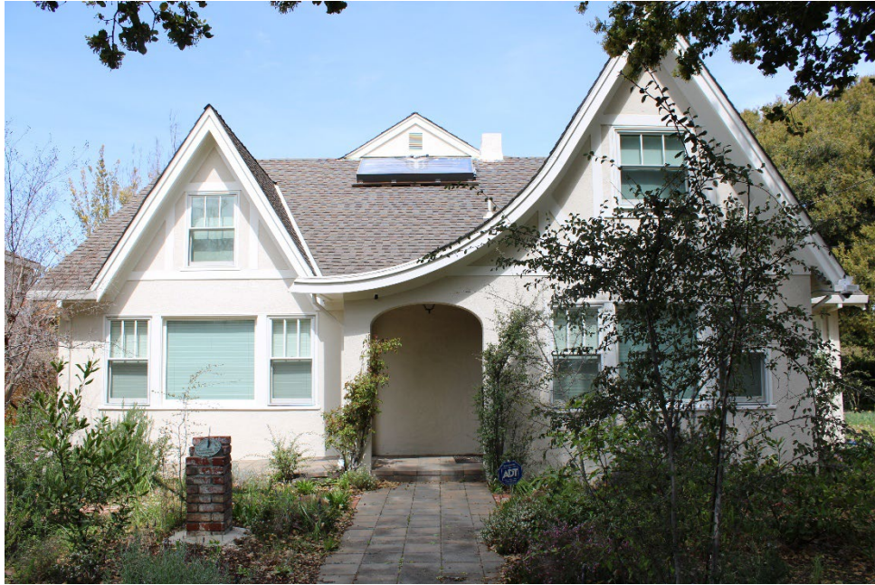
Figure 1. South elevation, facing north.
