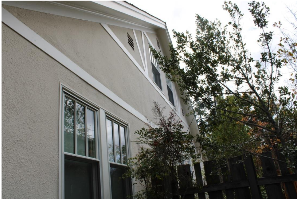
Figure 37. West elevation, facing southeast.
