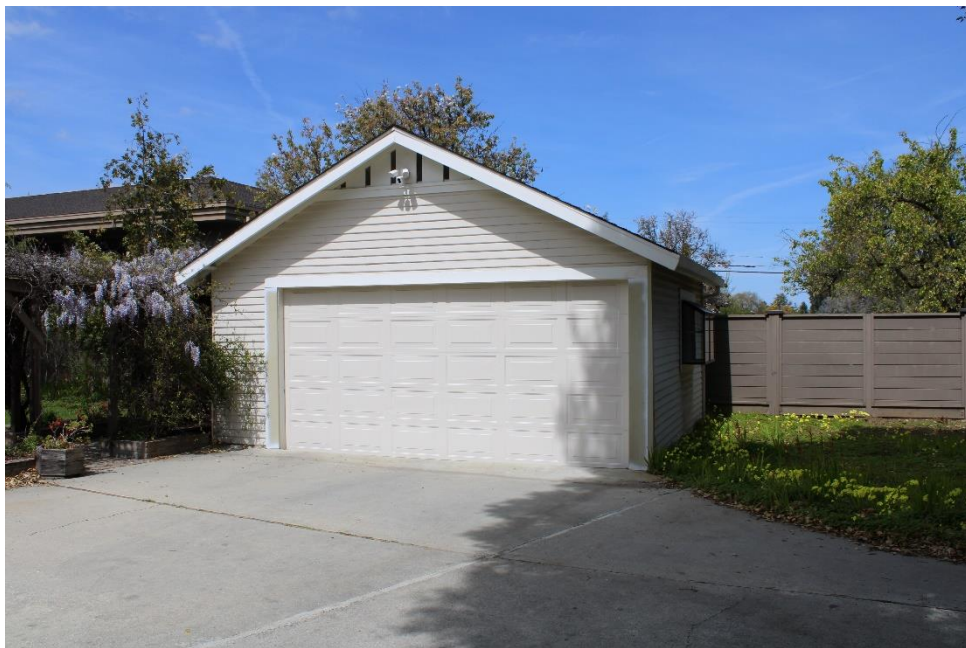
Figure 39. South elevation of detached garage, facing north.
