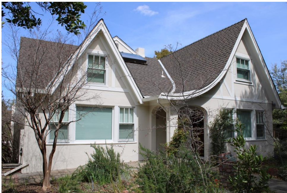
Figure 30. South elevation, facing northeast.
