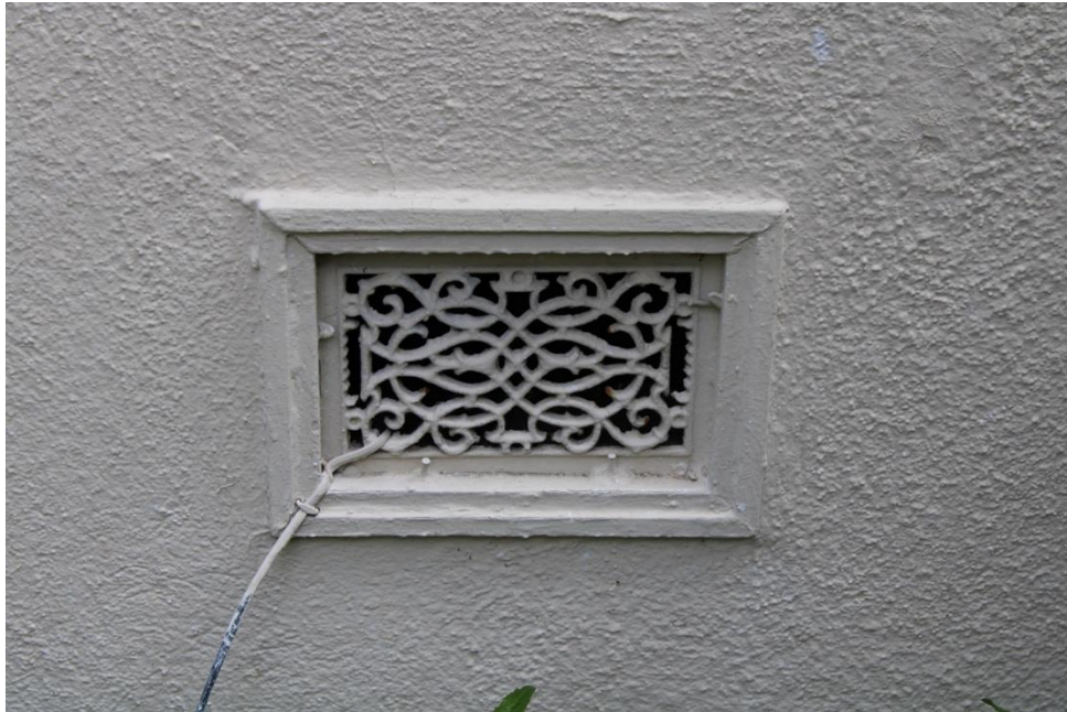
Figure 38. Cast-iron vent cover at the foundation.
