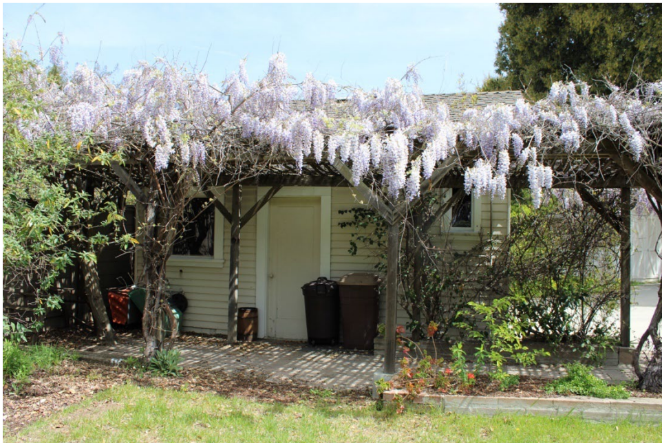
Figure 12. West elevation and trellis-covered walkway, facing east.
