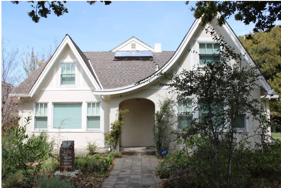
Figure 29. South elevation, facing north.
