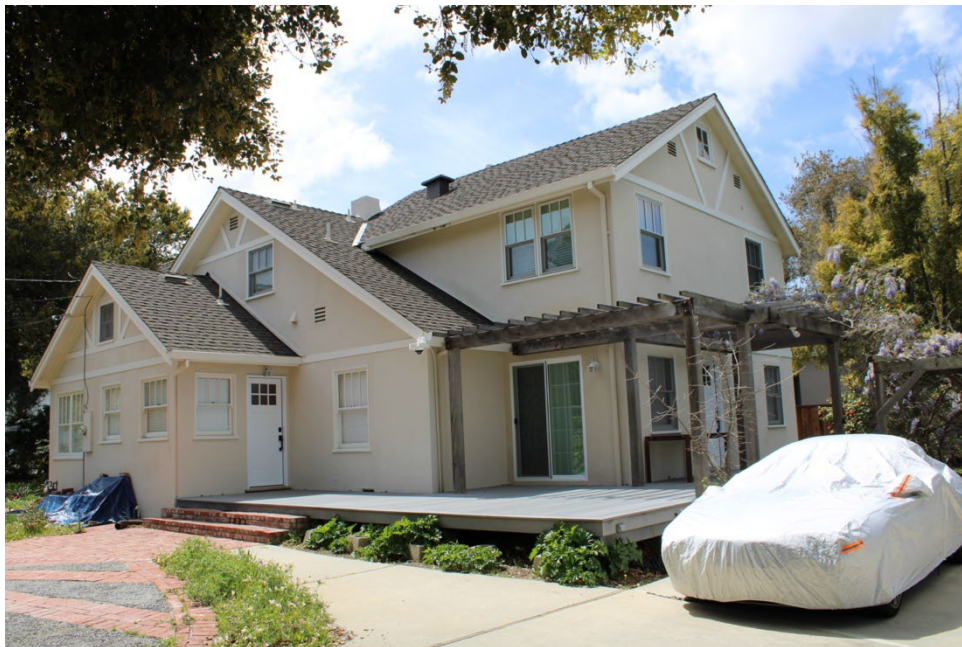
Figure 6. East elevation, facing southwest.
