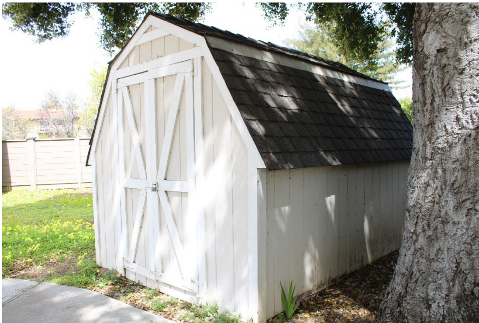
Figure 13. Photograph showing the double-entry doors along the southwest elevation (primary façade) of the ca. 1980 storage shed, facing north.
