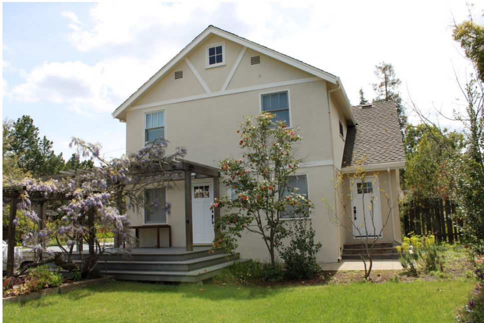
Figure 8. North elevation, facing south.
