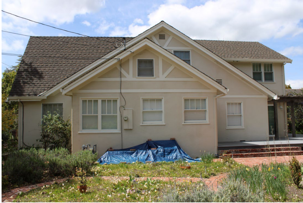
Figure 4. East elevation, facing west.
