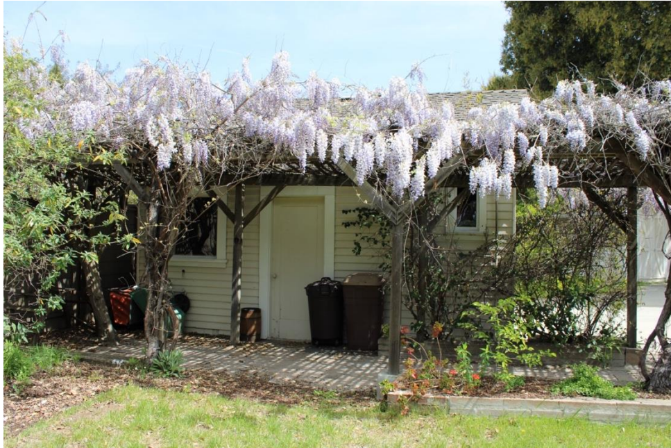
Figure 40. West elevation and trellis-covered walkway, facing east.
