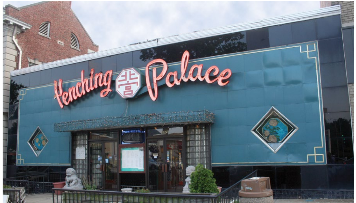
[11] (a) Some of the materials on the front of this historic building had been previously replaced, but the façade retained its essential distinctive features and design. (b) A vintage postcard of the building (far left) provided sufficient documentation to restore the façade to its historic 1945 appearance, using spandrel glass as a replacement for the original Carrara glass (c). Photo (b): Courtesy Kelsey & Associates.
