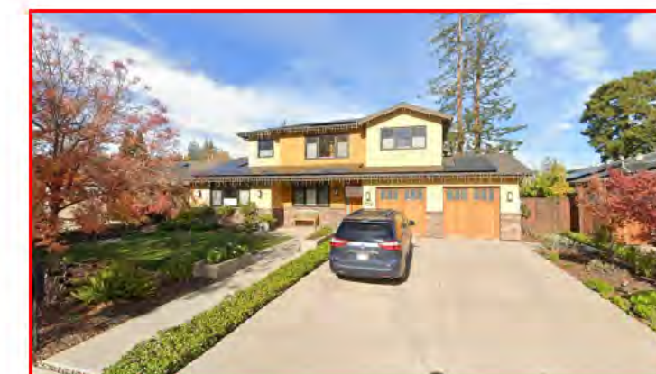
702 BENVENUE AVE. TWO STORY MATERIAL: STUCCO & STONE VENEER WALL AND COMPOSITION SHINGLE ROOF GARAGE: 2 CAR / PROJECTING FROM FRONT OF HOUSE FACE
