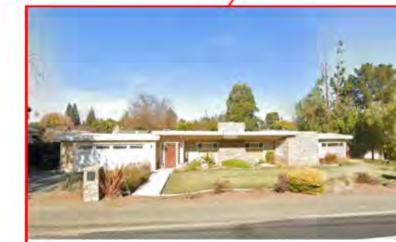
811 CUESTA DRIVE ONE STORY MATERIAL: STUCCO WALL AND TPO FLAT ROOF GARAGE: 2 CAR / RECESSED FROM HOUSE FRONT FACE
