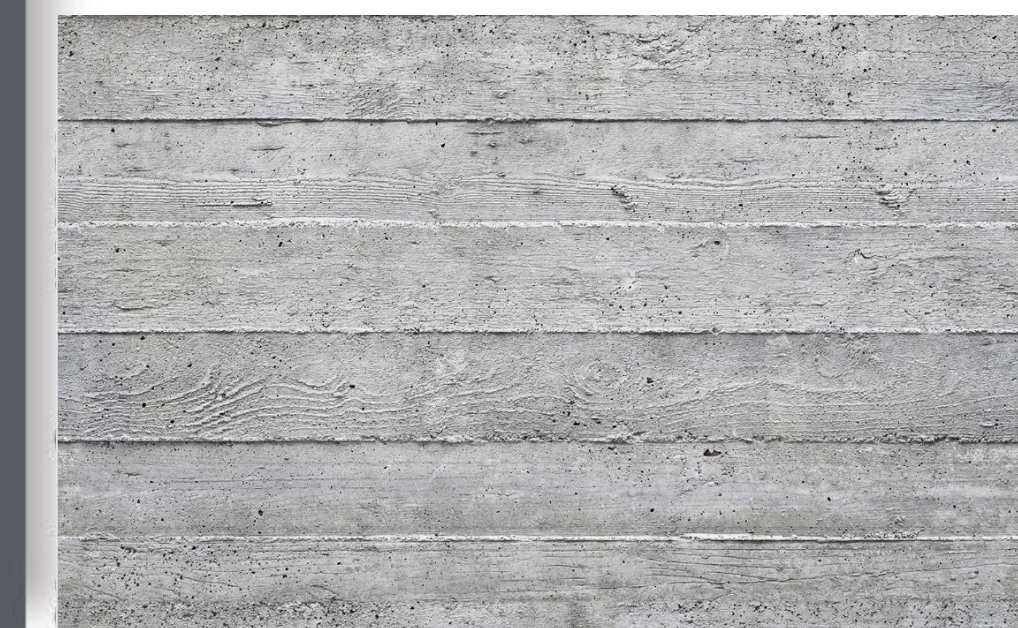
BOARD-FORM CONCRETE LANDSCAPE WALLS
