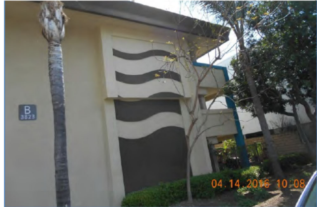
Figure 5: Although façade-mounted boxes are not preferred, this example from San Diego achieves integration with the structure.
