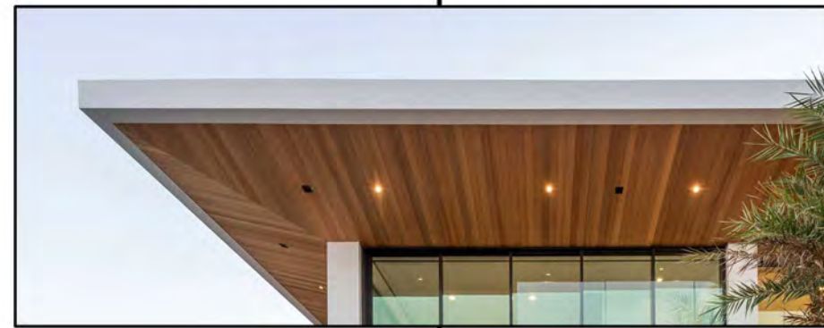
WOOD-LOOK BOARD SOFFIT AT UPPER ROOF OVERHANG
