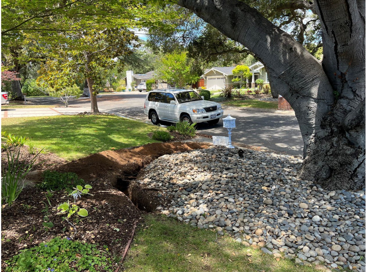
Location of exploratory trenching around Tree # 5
