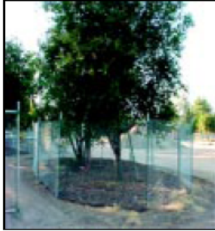
IMAGE 2.15-1 Tree Protection Fence at the Dripline
