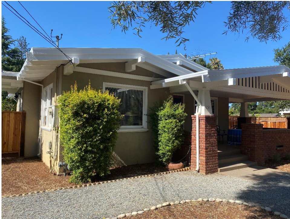
Figure 24. South elevation, facing north.
