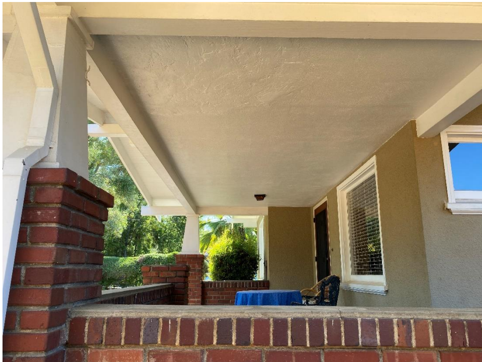
Figure 25. Photograph showing the front porch, facing west.
