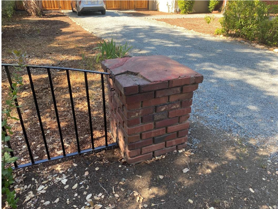
Figure 36. Photograph showing a concrete pillar and contemporary iron gate along the primary façade, facing north.
