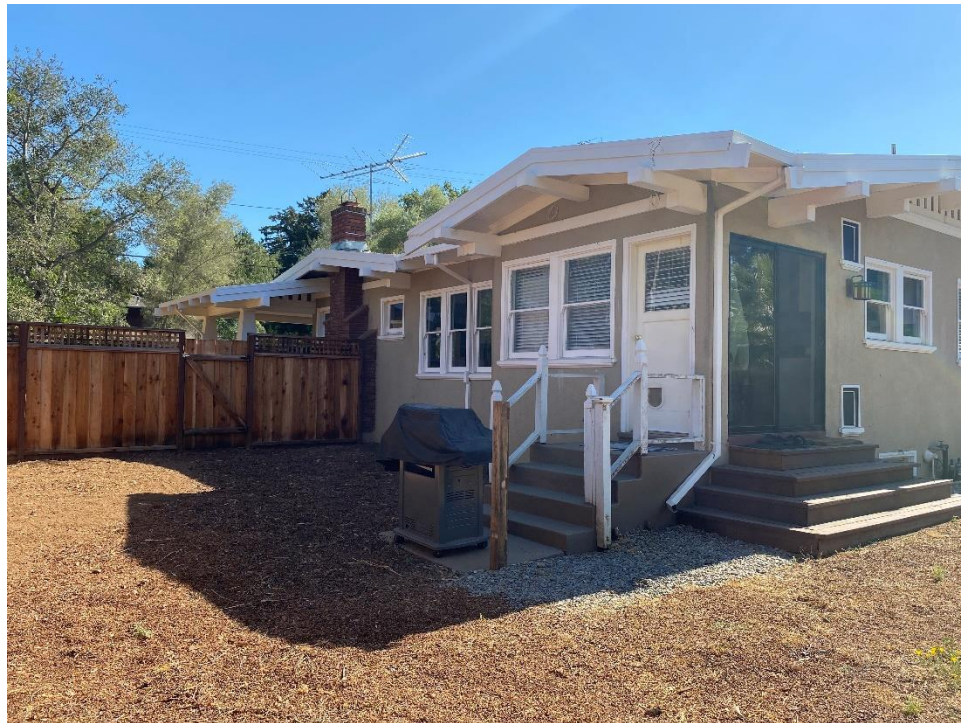
Figure 28. Photograph showing the east elevation, facing southwest.
