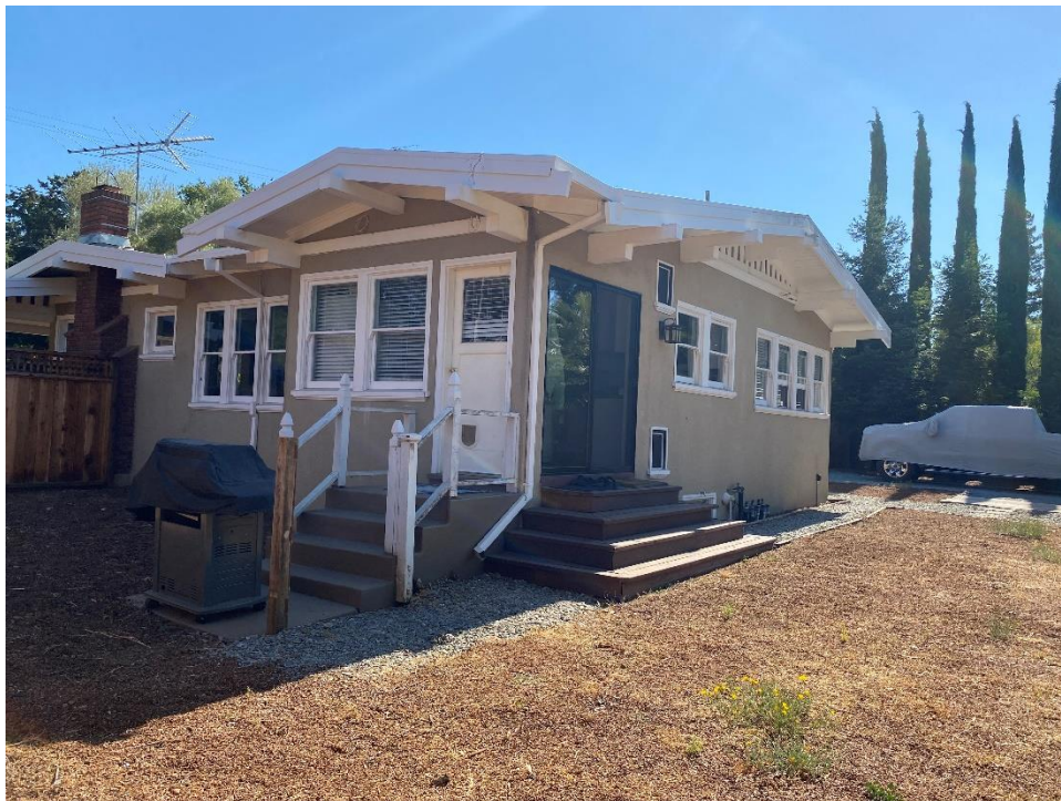
Figure 29. Photograph showing the north elevation rear roof gable and decorative vertical wood boards along the gable, facing southwest.
