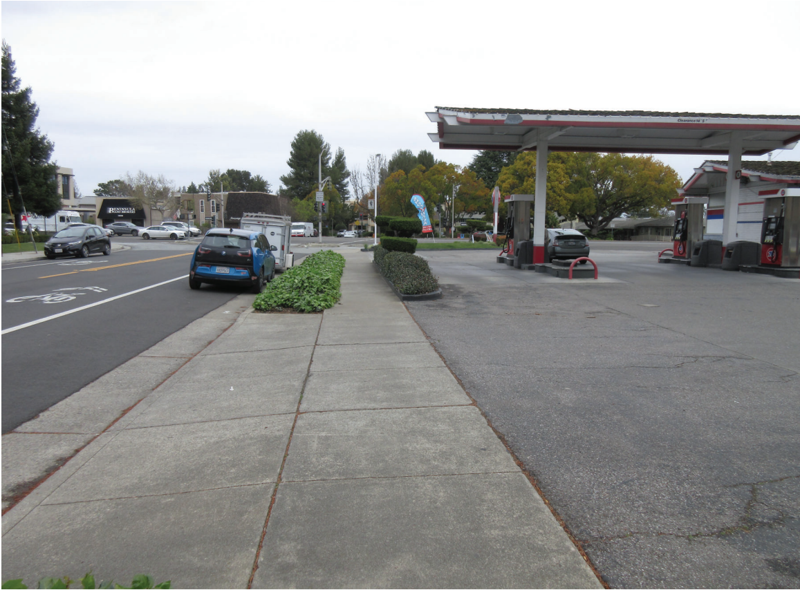
Photo 3: Viewing northeast along the project frontage on Los Altos Avenue from the southwest corner of the site.
