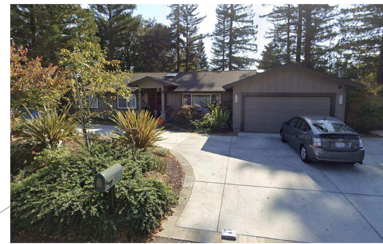
340 HAWTHORNE AVE, LOS ALTOS, CA 94022 ONE-STORY SINGLE FAMILY HOUSE
