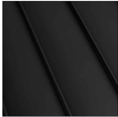
STANDING SEAM METAL ROOF INTERLOCK, BLACK
