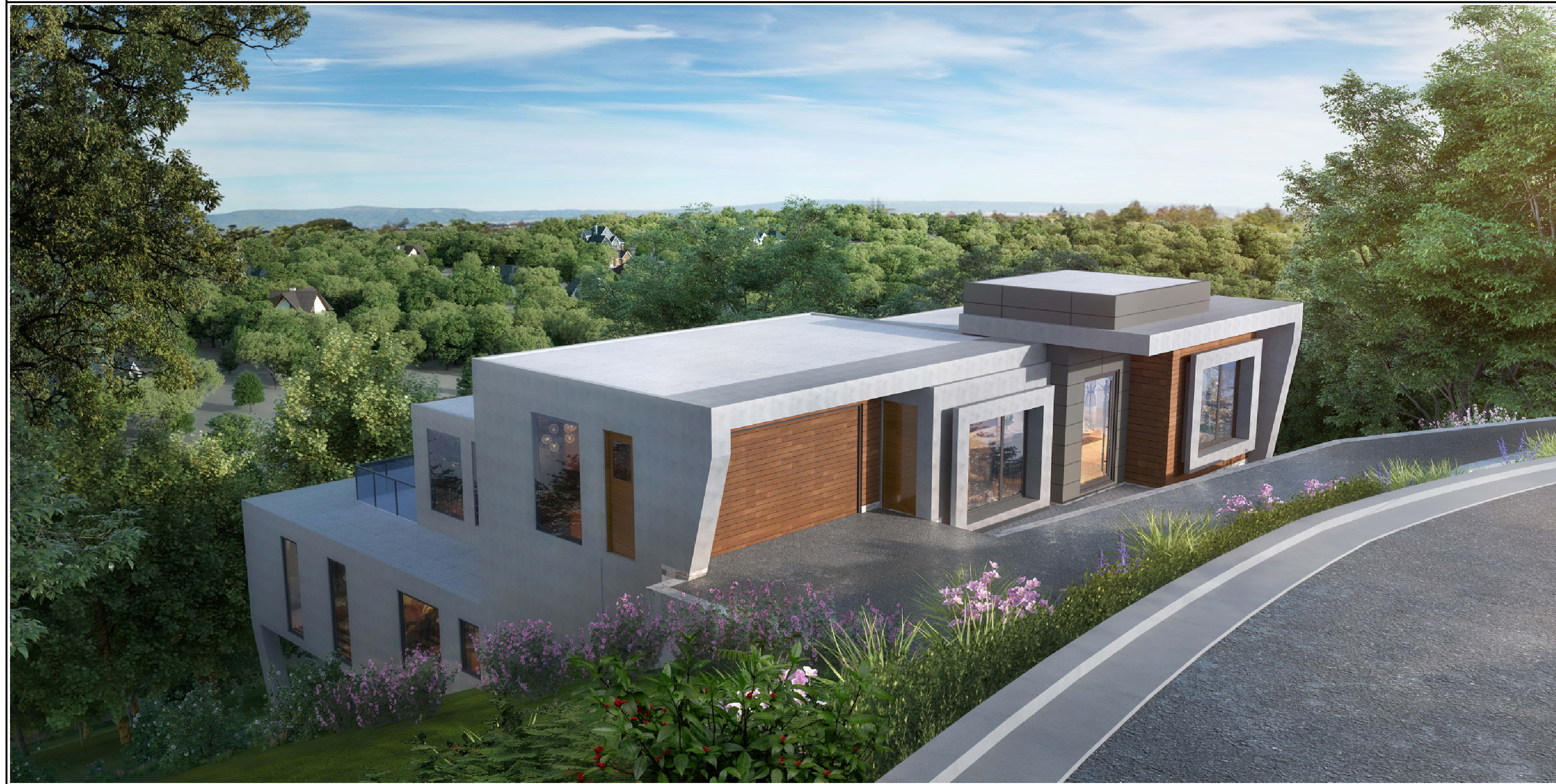
③ VIEW FROM STREET GOING DOWNHILL
