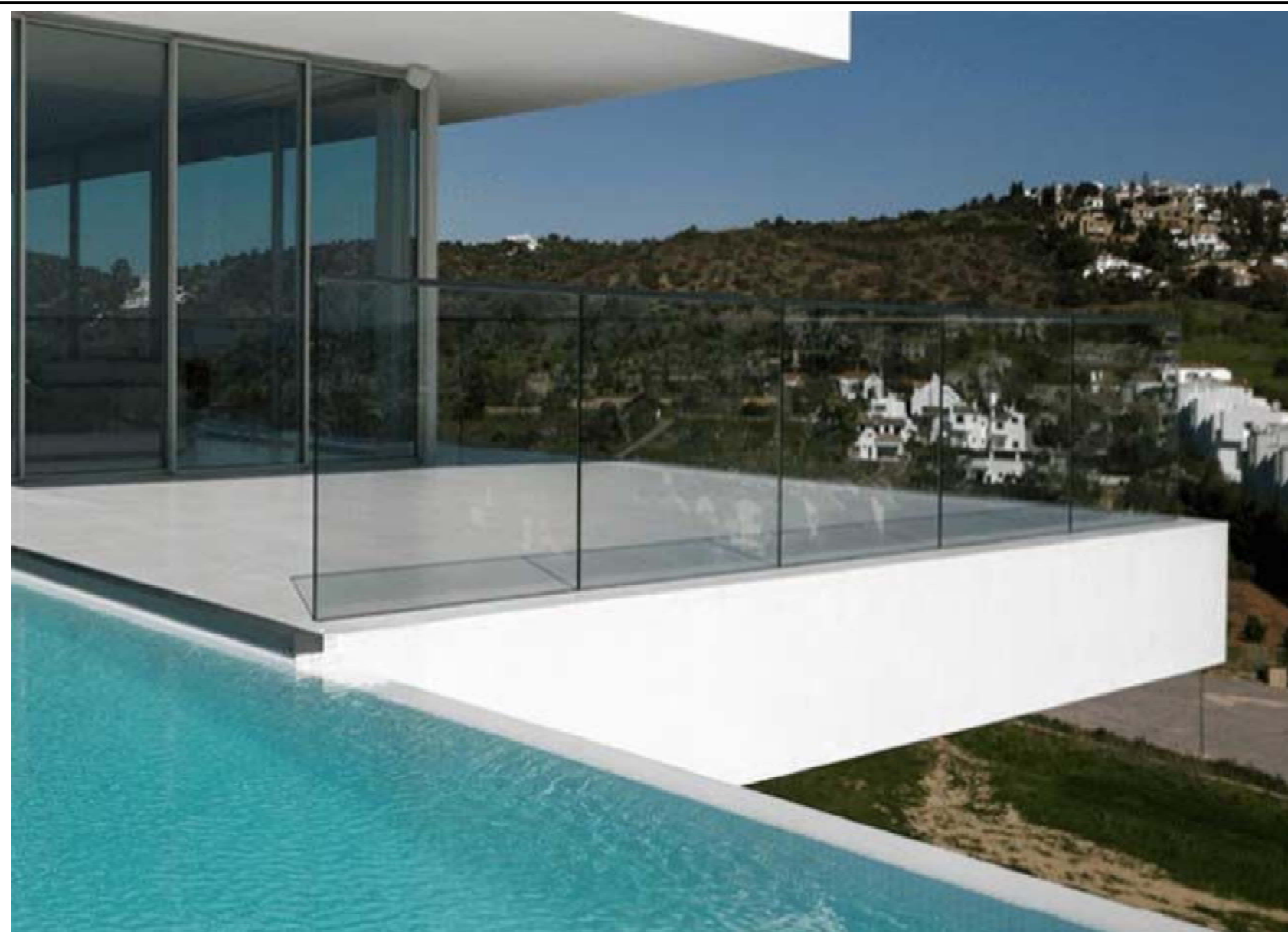
④ GLASS RAILING
