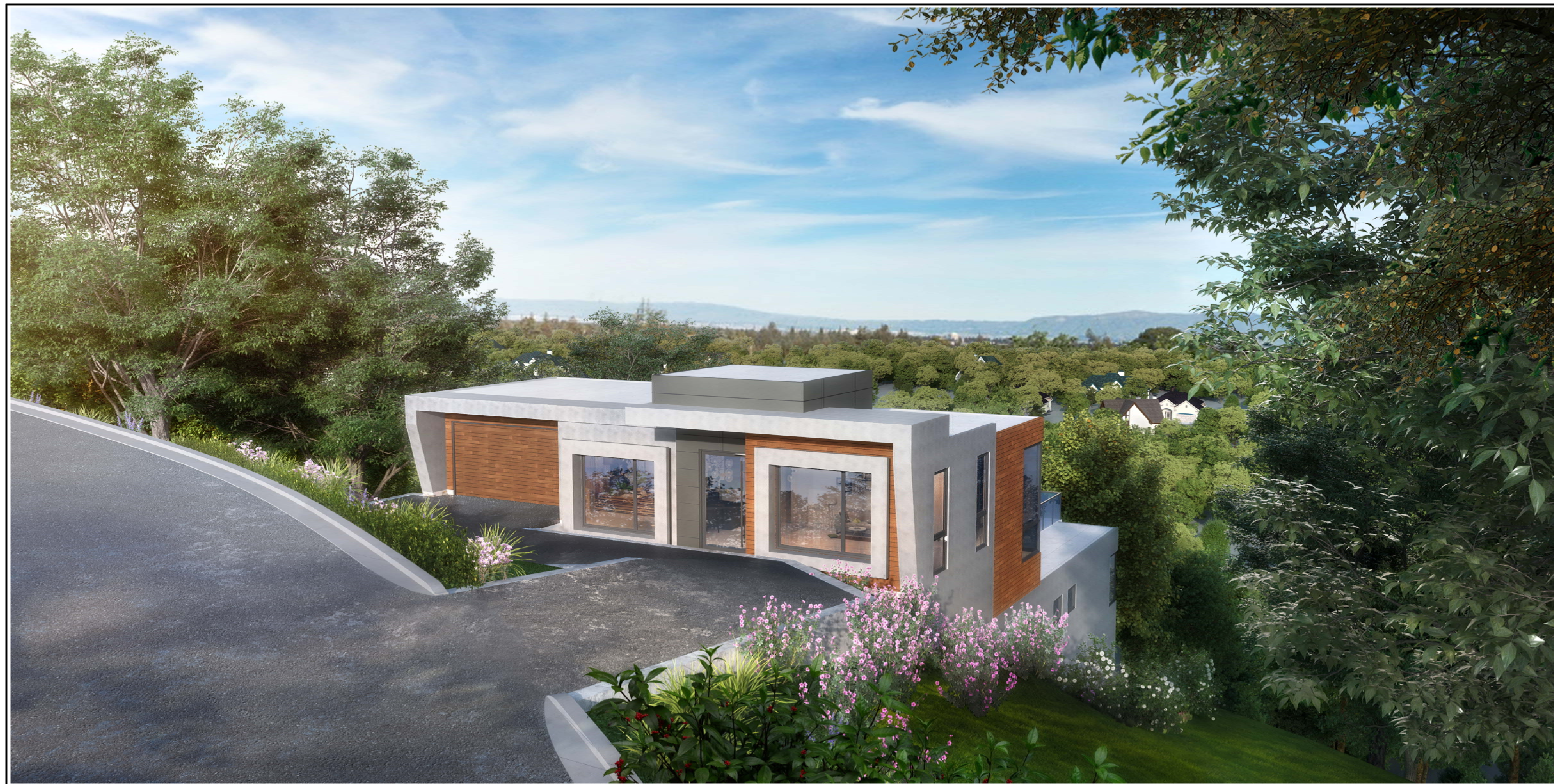
② VIEW FROM STREET GOING UPHILL
