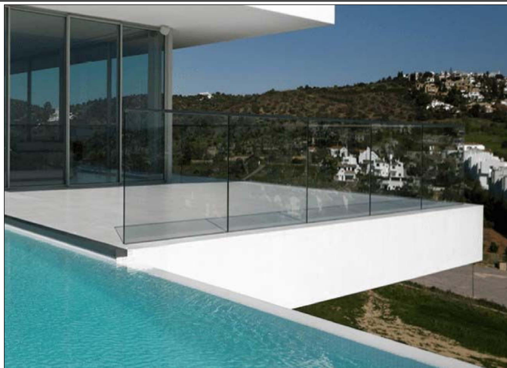
④ GLASS RAILING
