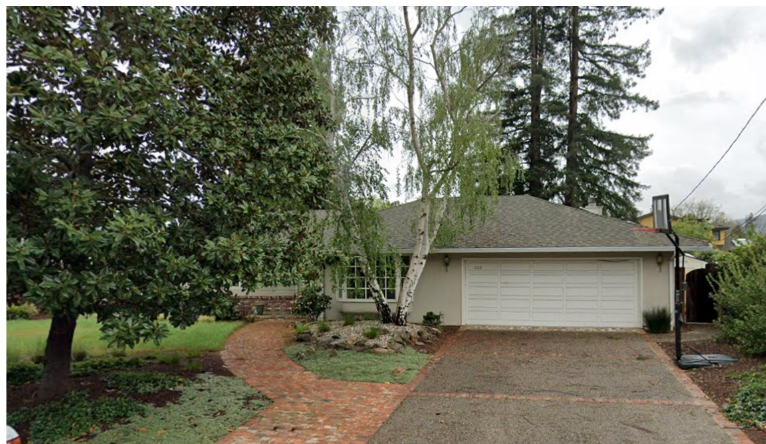
622 BENVENUE AVE 1-STORY HOUSE
