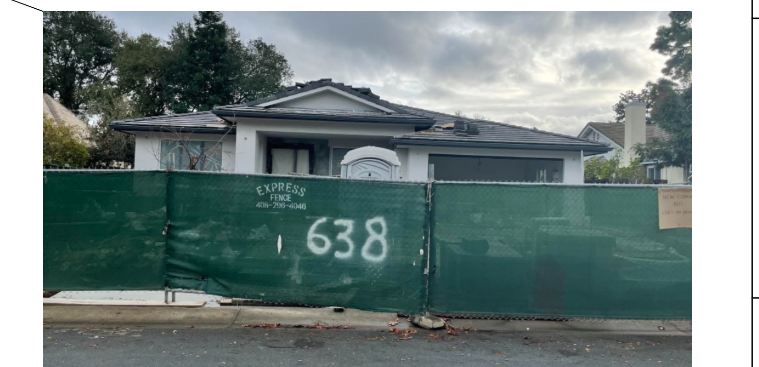
638 BENVENUE AVE (IN CONSTRUCTION) 1-STORY HOUSE
