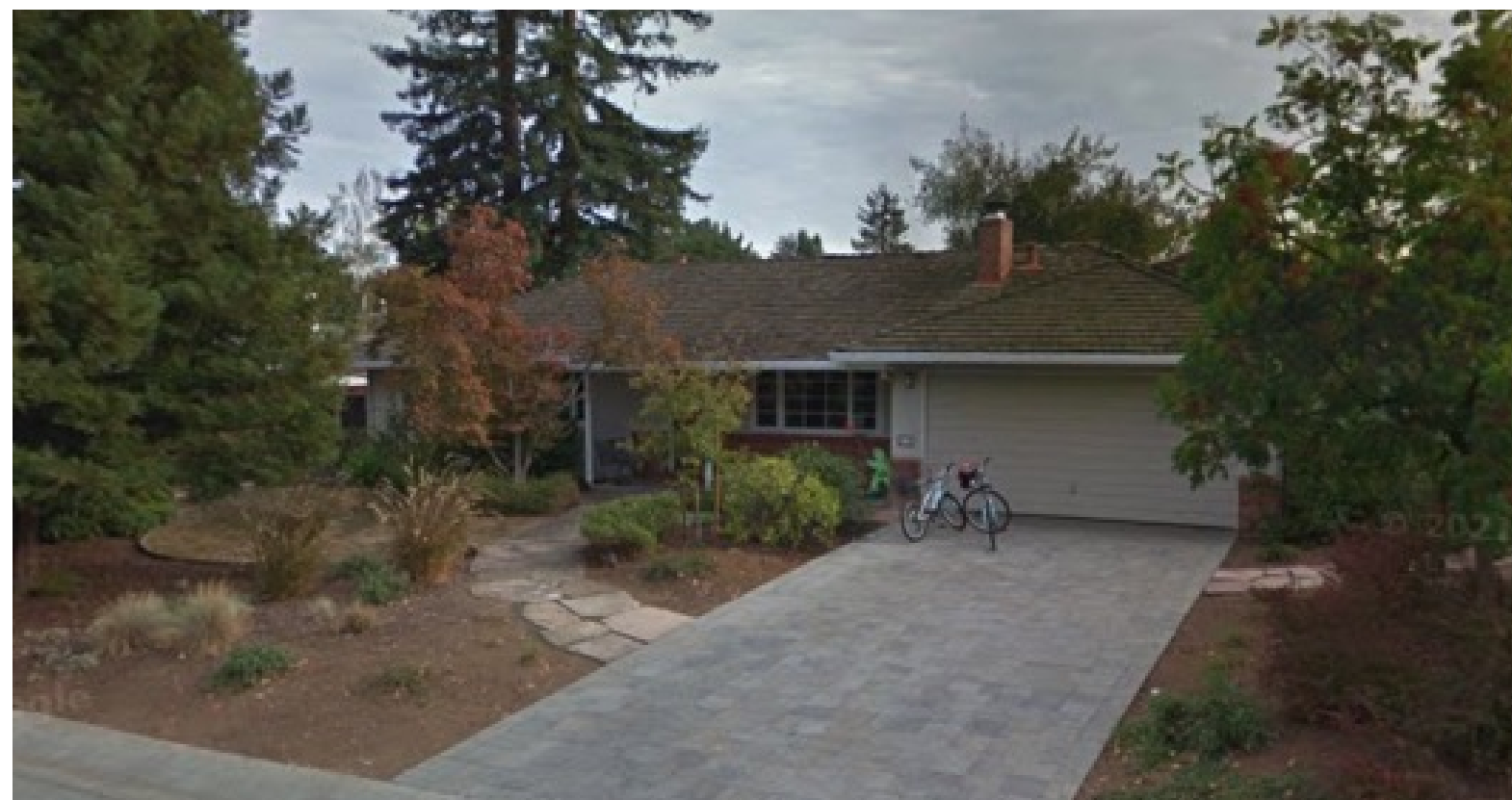
618 BENVENUE AVE 1-STORY HOUSE
