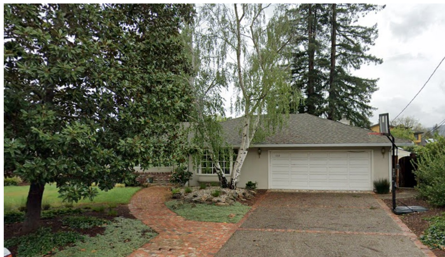
622 BENVENUE AVE 1-STORY HOUSE
