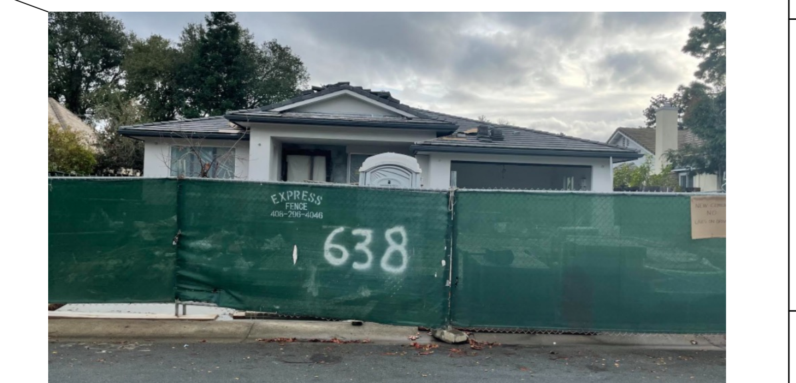
638 BENVENUE AVE (IN CONSTRUCTION) 1-STORY HOUSE
