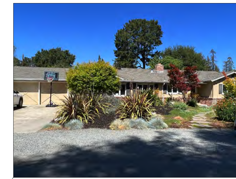
110 OSAGE AVENUE HOUSE STYLE: RANCH NUMBER OF STORIES: 1 EXTERIOR MATERIALS: BOARD & BATTEN & BRICK ROOF STYLE: GABLE ROOF MATERIAL: COMP SHINGLE
