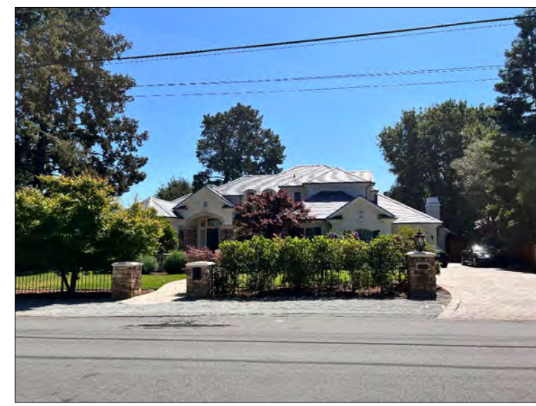
111 S GORDON WAY HOUSE STYLE: NEO FRENCH NUMBER OF STORIES: 2 EXTERIOR MATERIALS: STUCCO & STONE ROOF STYLE: HIP ROOF MATERIAL: COMP SHINGLE
