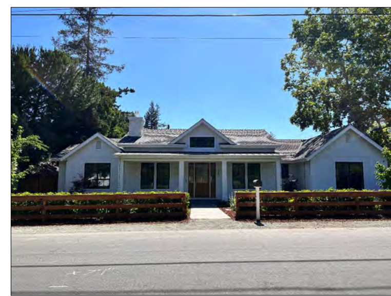
141 S GORDON WAY HOUSE STYLE: MODERN NUMBER OF STORIES: 1 EXTERIOR MATERIALS: BOARD & BATTEN ROOF STYLE: GABLE ROOF MATERIAL: COMP SHINGLE & STANDING SEAM
