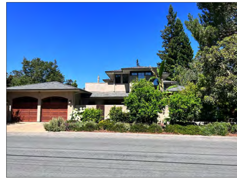
284 FRANCES DRIVE HOUSE STYLE: MODERN NUMBER OF STORIES: 2 EXTERIOR MATERIALS: STUCCO ROOF STYLE: HIP & VALLEY ROOF MATERIAL: COMP SHINGLE
