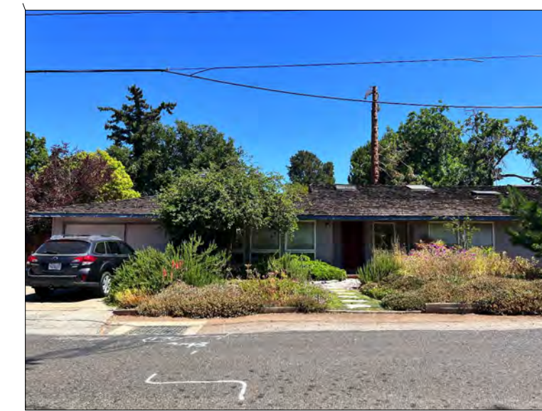
321 HILLVIEW AVENUE HOUSE STYLE: RANCH NUMBER OF STORIES: 1 EXTERIOR MATERIALS: CLAPBOARD ROOF STYLE: HIP ROOF MATERIAL: SHAKE
