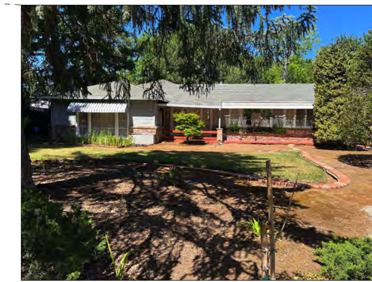
124 OSAGE AVENUE HOUSE STYLE: RANCH NUMBER OF STORIES: 1 EXTERIOR MATERIALS: CLAPBOARD & BRICK ROOF STYLE: GABLE ROOF MATERIAL: COMP SHINGLE
