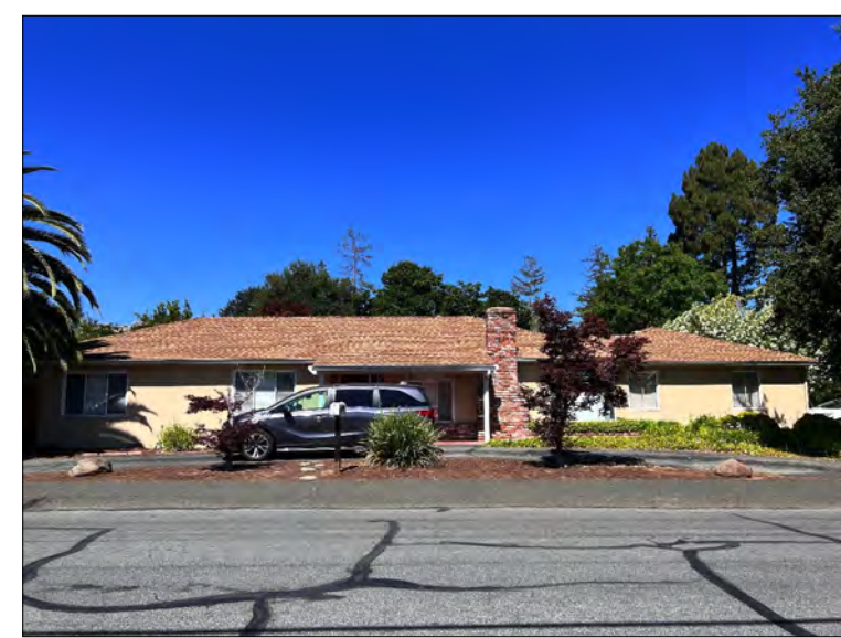
160 S GORDON WAY HOUSE STYLE: RANCH NUMBER OF STORIES: 1 EXTERIOR MATERIALS: STUCCO & BRICK ROOF STYLE: HIP ROOF MATERIAL: COMP SHINGLE
