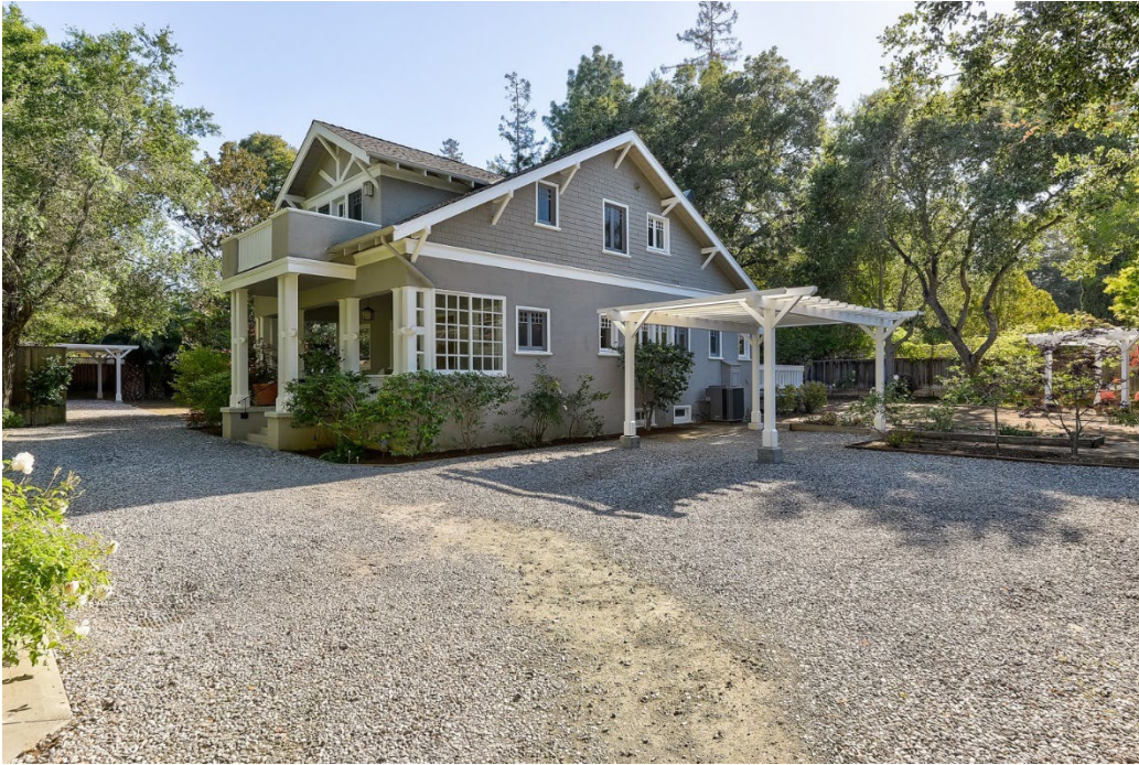
Photograph 4 236 Eleanor Avenue, Los Altos View: The north side façade showing the window alteration to fill the side of the porch and the second level gable. A carport is under the pergola structure and the entrance to the rear of the house..
