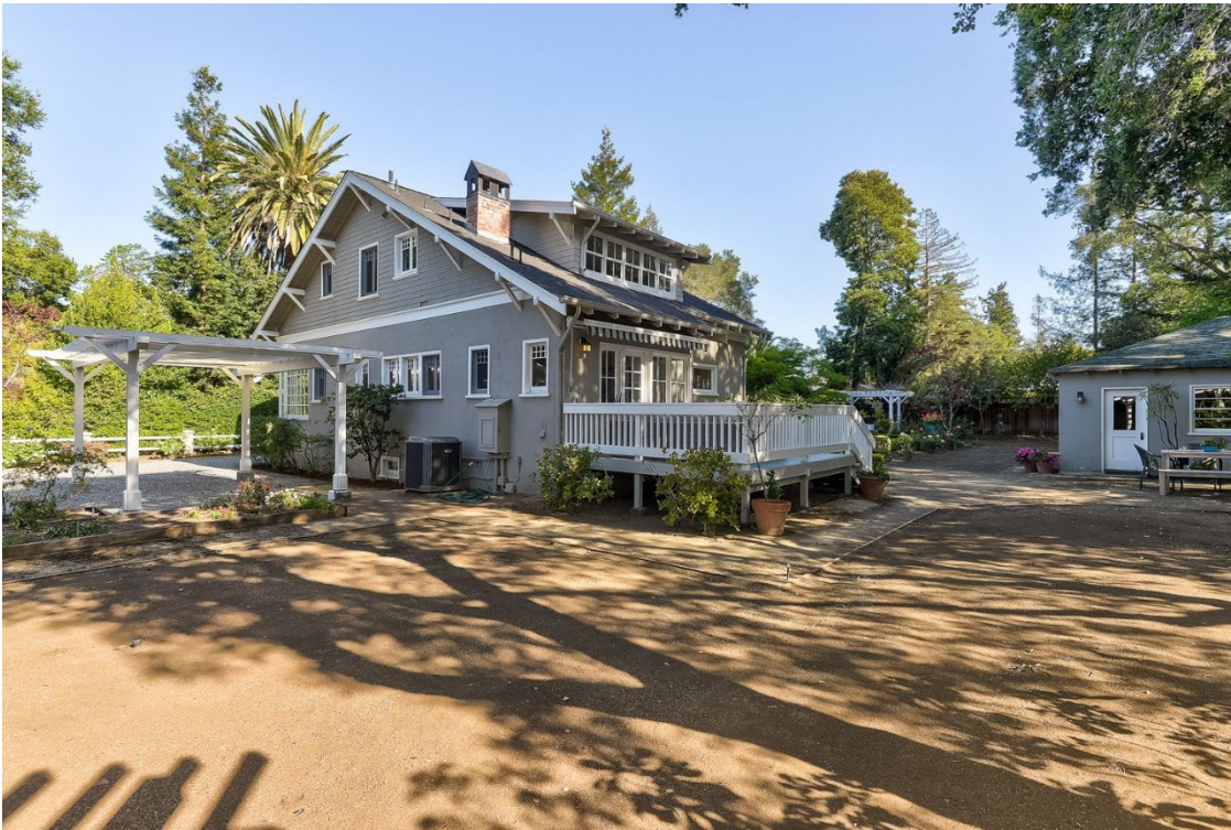
Photograph 6 236 Eleanor Avenue, Los Altos View: Rear and north side showing the rear additions and deck addition. A shed is behind the house and the carport on the left (north) side.
