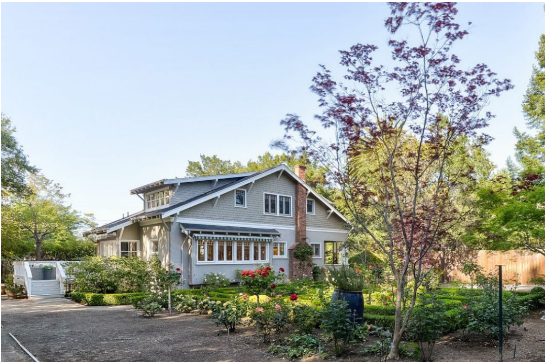
Photograph 5 236 Eleanor Avenue, Los Altos View: Rear façade showing the pop out addition to the original design. The view shows the shed dormer on the rear second level.
