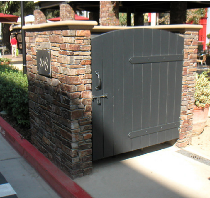
Use of materials and colors helps minimize appearance of a centralized trash enclosure.
