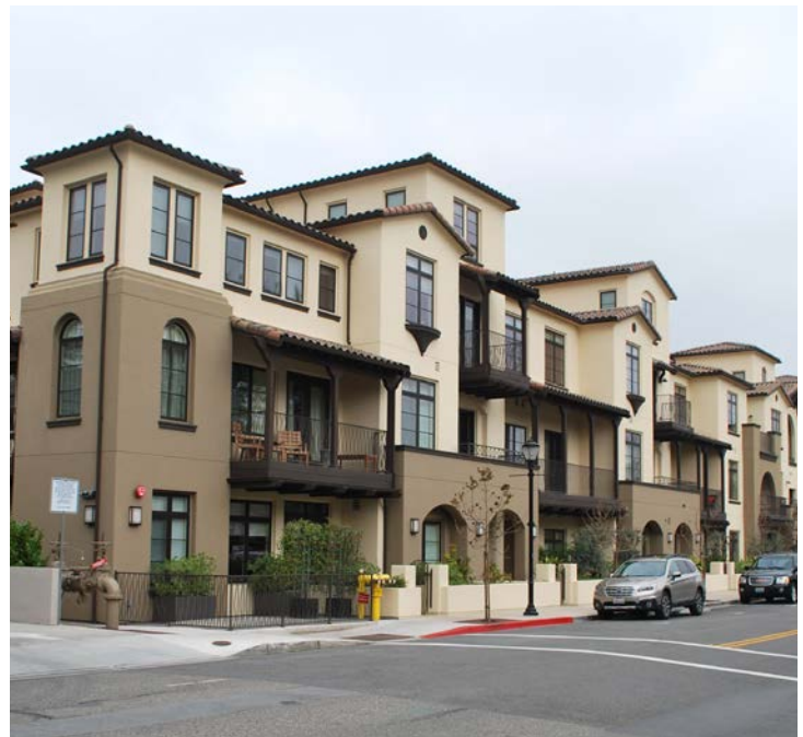
Existing residential development incorporates setbacks, articulation, and features that enhance the overall design.
