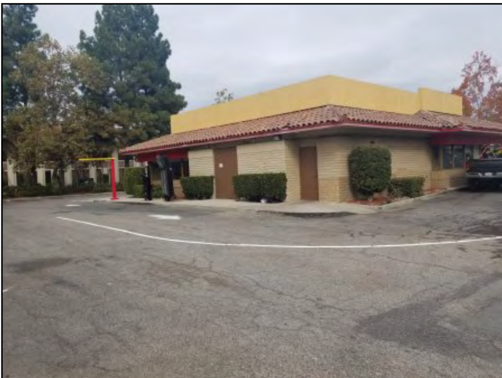
30 : View of the property to the north of the site.
