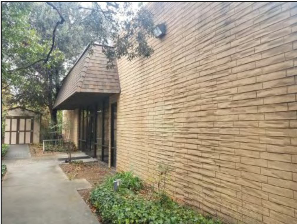
6 : View of the southern side of the site building.
