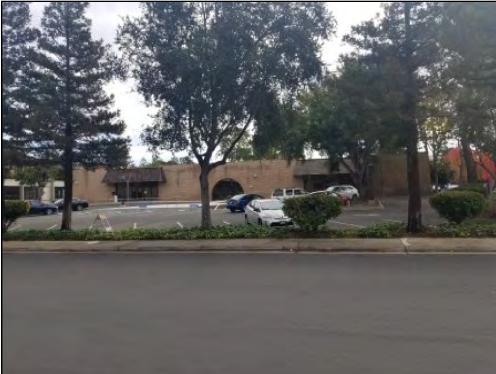
29 : View of the property to the east of the site.
