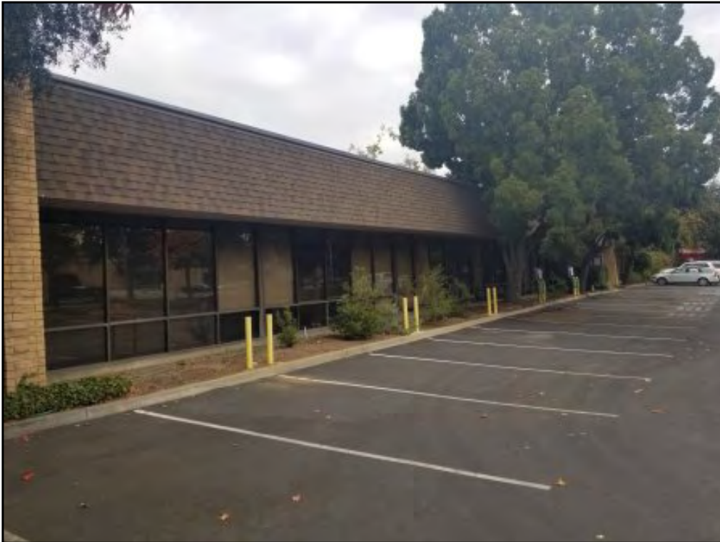
5 : View of the eastern side of the site building.
