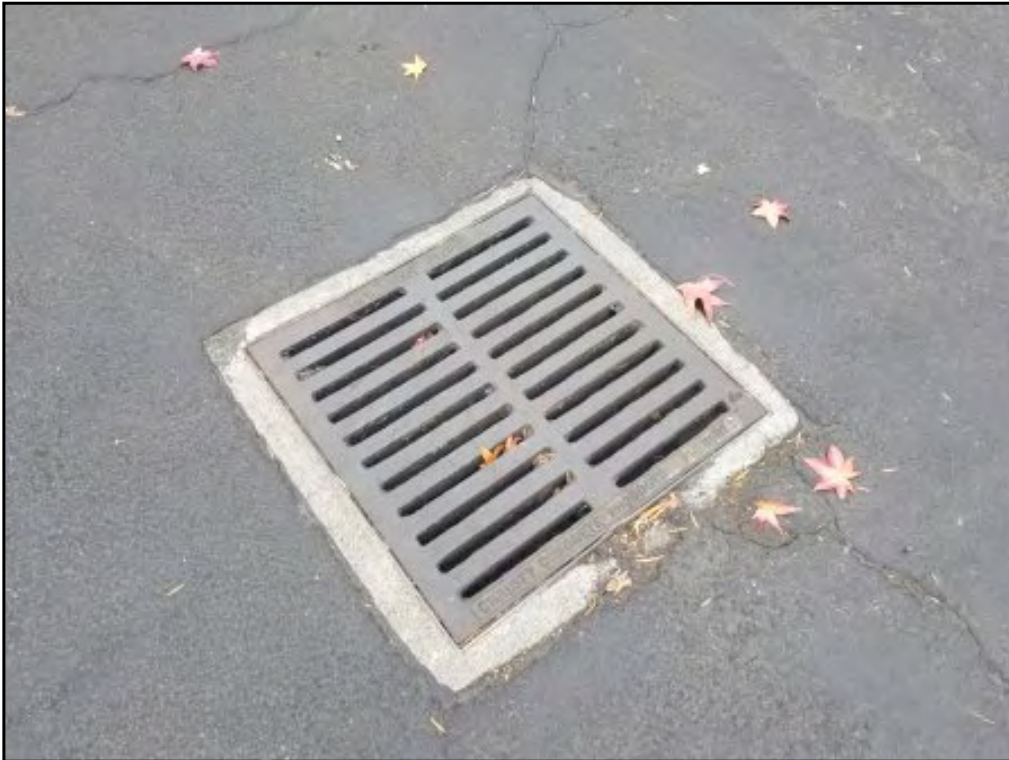
25 : View of a storm drain in the parking lot.
