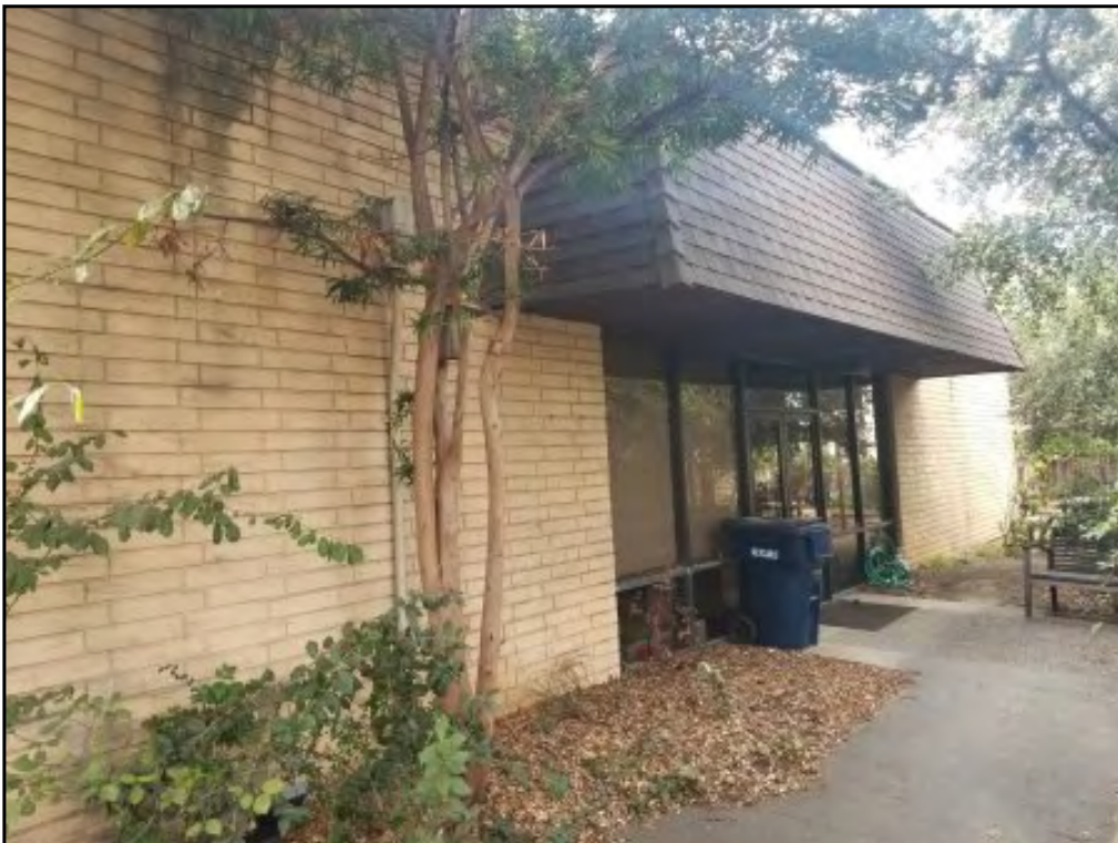
8 : View of the northern side of the site building.
