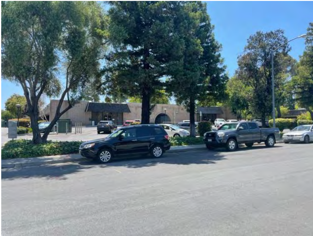
PHOTO #2. VIEW OF ADJACENT PARCEL TO EAST AND PROPERTY BUILDING.
