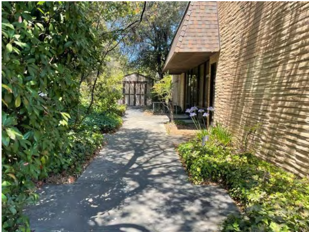
PHOTO #6. VIEW OF EXTERIOR AREAS ALONG SOUTHERN SIDE OF BUILDING.
