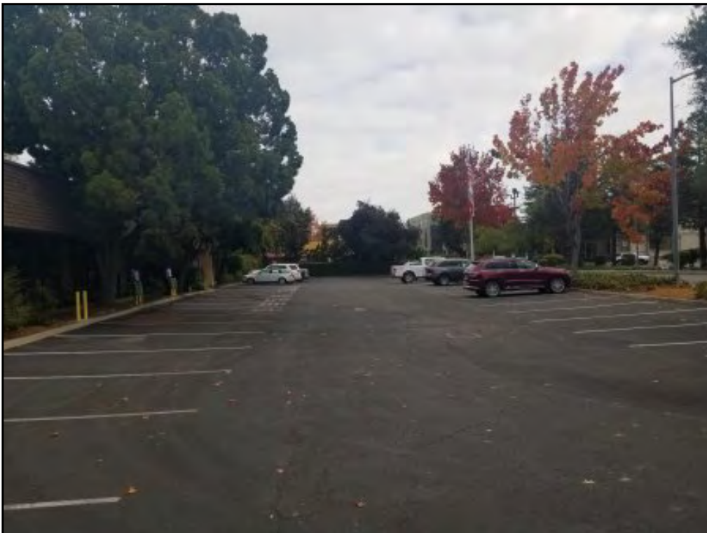
10 : View of the site parking lot, facing north.
