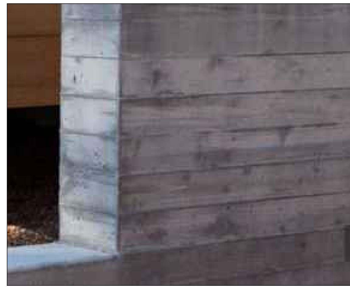
BOARD FORMED CONCRETE
