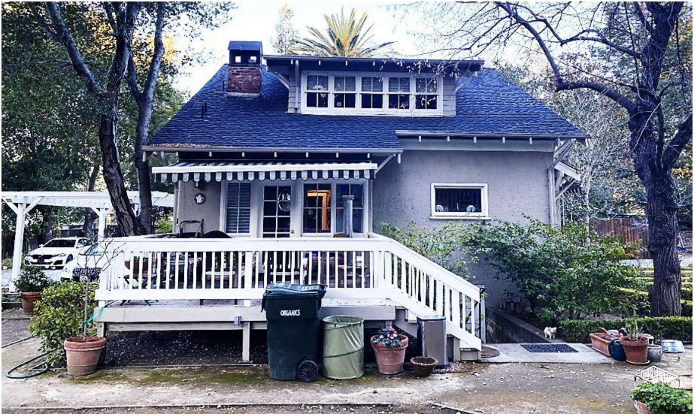
Photograph 7 236 Eleanor Avenue, Los Altos
