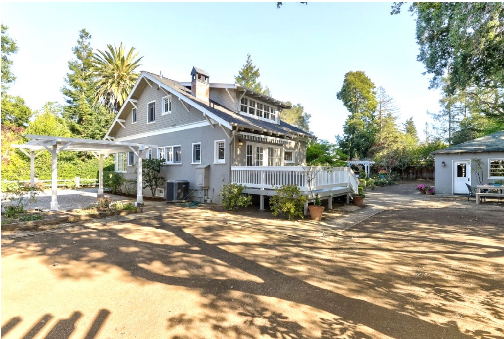
Photograph 6 236 Eleanor Avenue, Los Altos View: Rear and north side showing the rear and deck additions. A large shed dormer appears to be an addition that is out of proportion with the style and original dormer on the front façade. A contemporary shed is behind the house.
