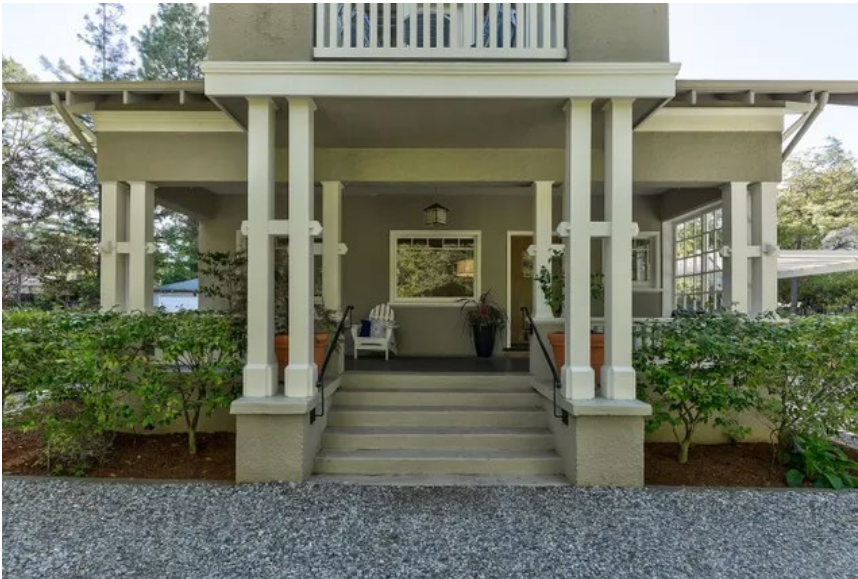
Photograph 3 236 Eleanor Avenue, Los Altos
