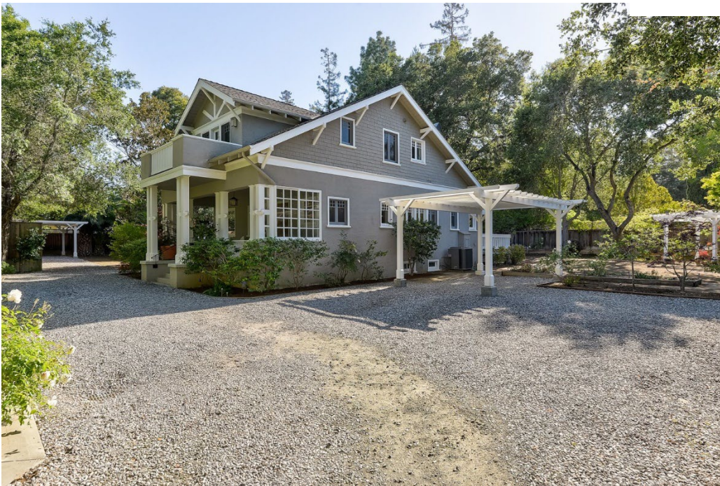
Photograph 4 236 Eleanor Avenue, Los Altos
