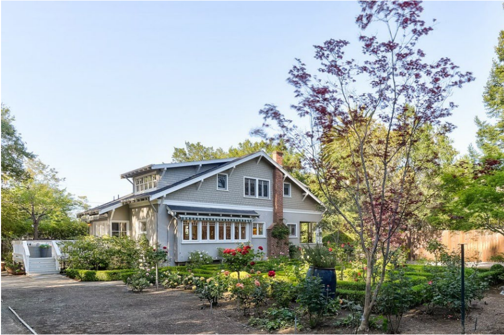
Photograph 5 236 Eleanor Avenue, Los Altos View: West and rear façades showing the pop-out addition to the original design. The view shows the shed dormer addition on the rear roof, creating a second level.
