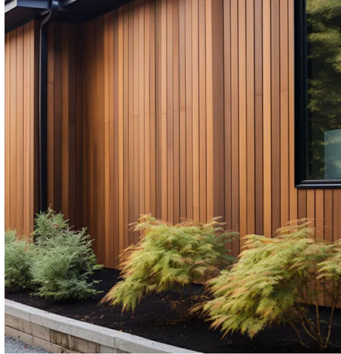
VERTICAL WOOD SIDING, STAINED
