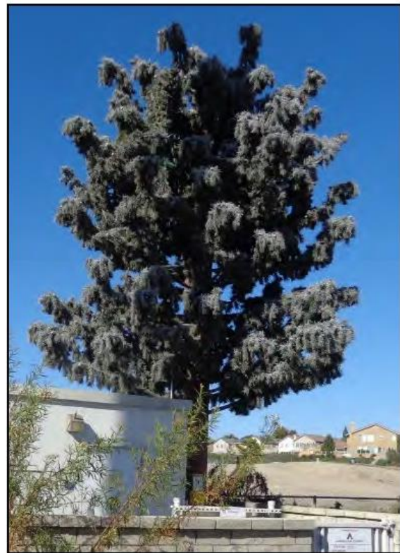
Figure 6: In this example, antennas are concealed by the faux "mono-pine."
