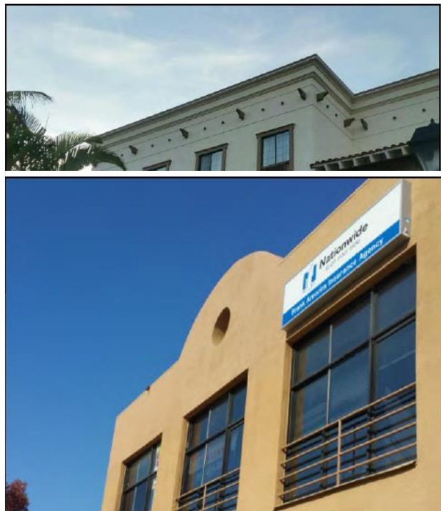
Figure 2: Antennas are concealed behind the circular element.
