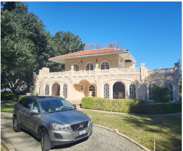
Figure 2. Primary (south) façade of main house, view northwest, 2024.
