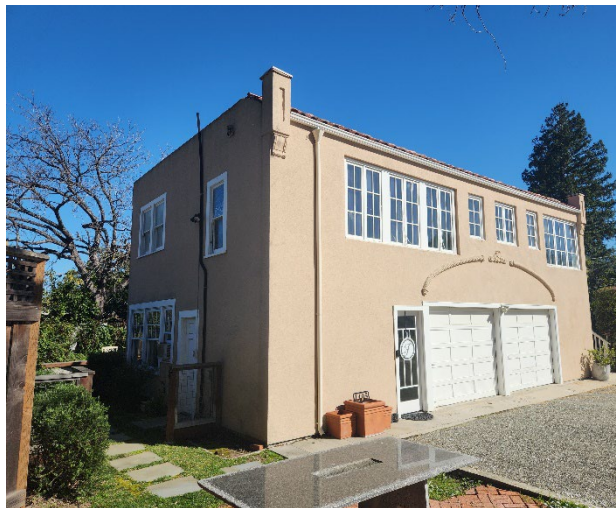
Figure 3. Side (west, left) and primary (south, right) facades of garage apartment, view northeast, 2024.
