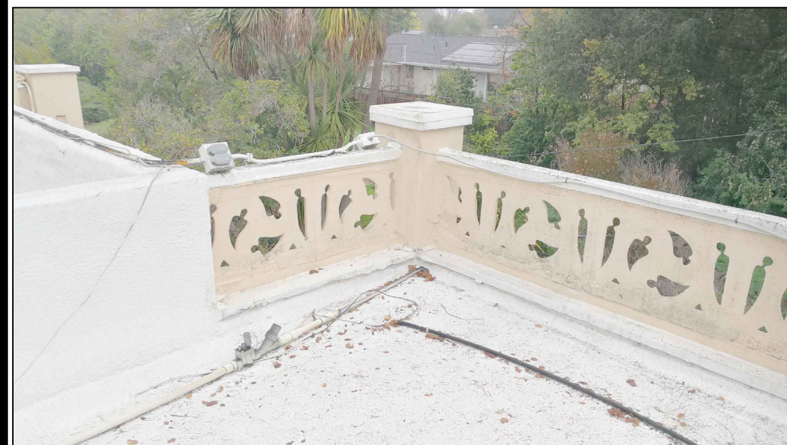
IMAGE C: @ UPPER BALCONY PARAPET
