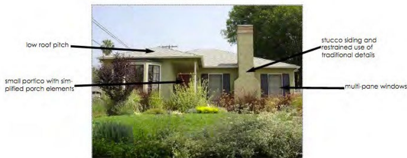
Figure 6. Minimal Traditional style markers as shown on a Minimal Traditional home in Glendale, California (Glendale Design Guidelines for Residential Buildings in Adopted Historic Districts) 5
