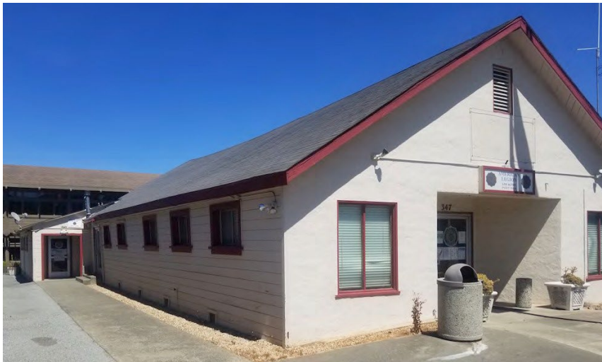
Figure 9. Oblique view of southwest elevations looking north (W. Bassett, 2021)
