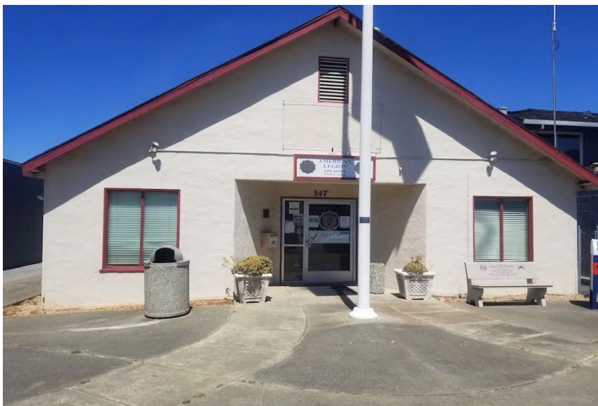
Figure 8. Exterior, south elevation, showing current hardscape (W. Bassett, 2021)
