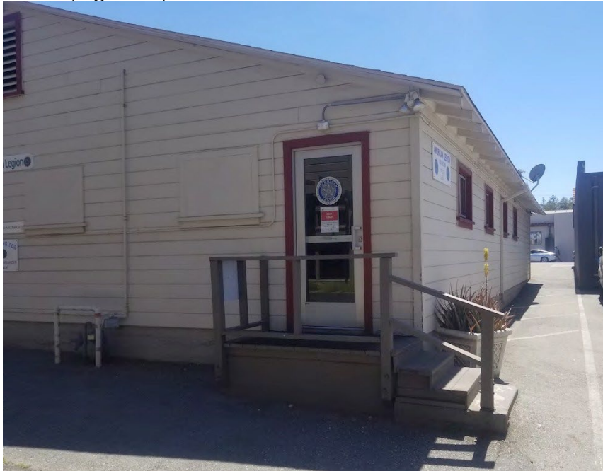
Figure 11. Oblique view of rear (north) elevation, looking south (W. Bassett, 2021)
