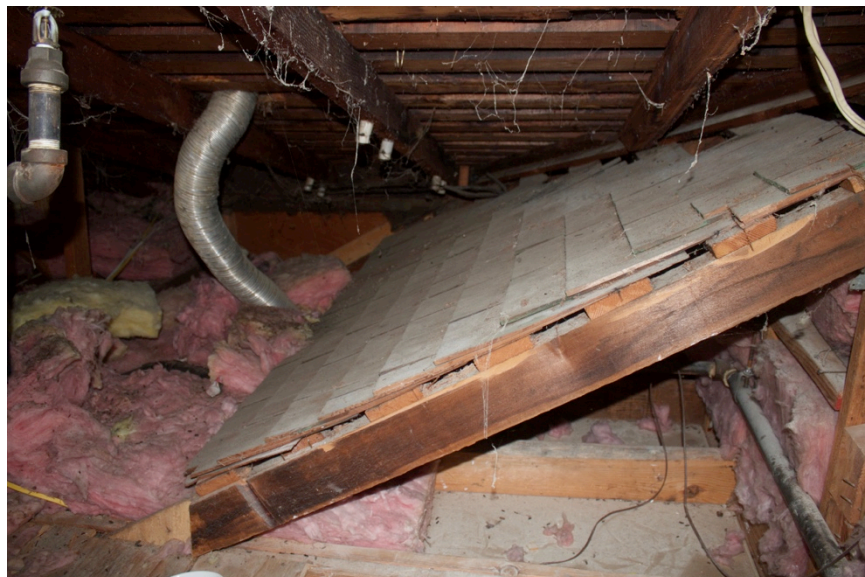
Figure 24: Picture of original cottage's roof inside the attic of the Costello House (Garavaglia Architecture, 2022)
