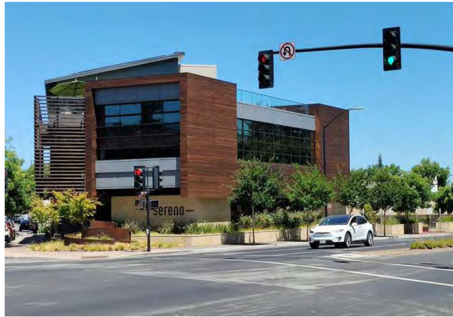
[1] SERENO BUILDING - 467 1ST ST.
