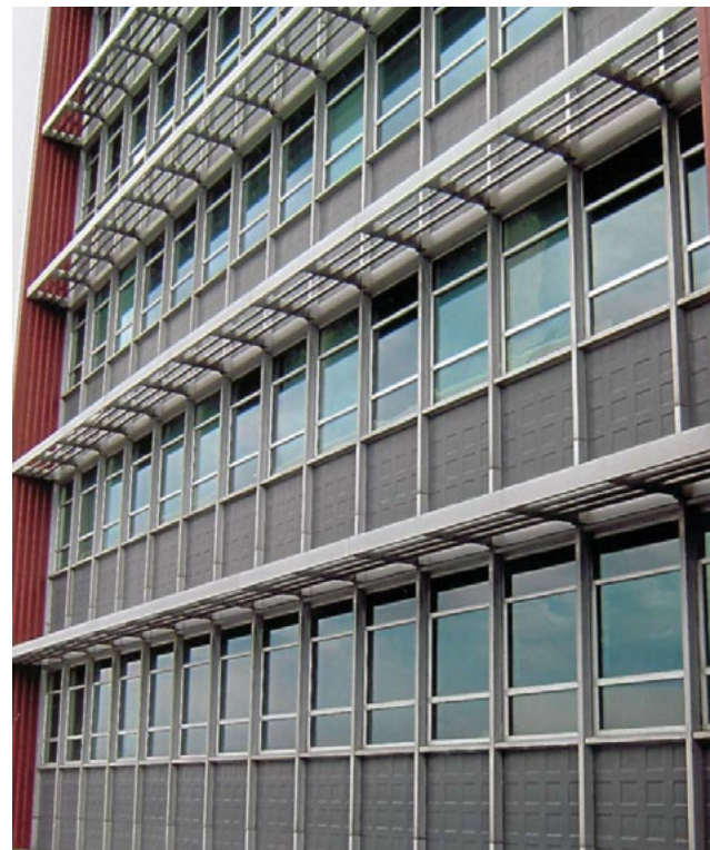
[12] This historic curtain wall features a distinctive variety of panel types which must be repaired or replicated in a restoration project if any are damaged or missing.
