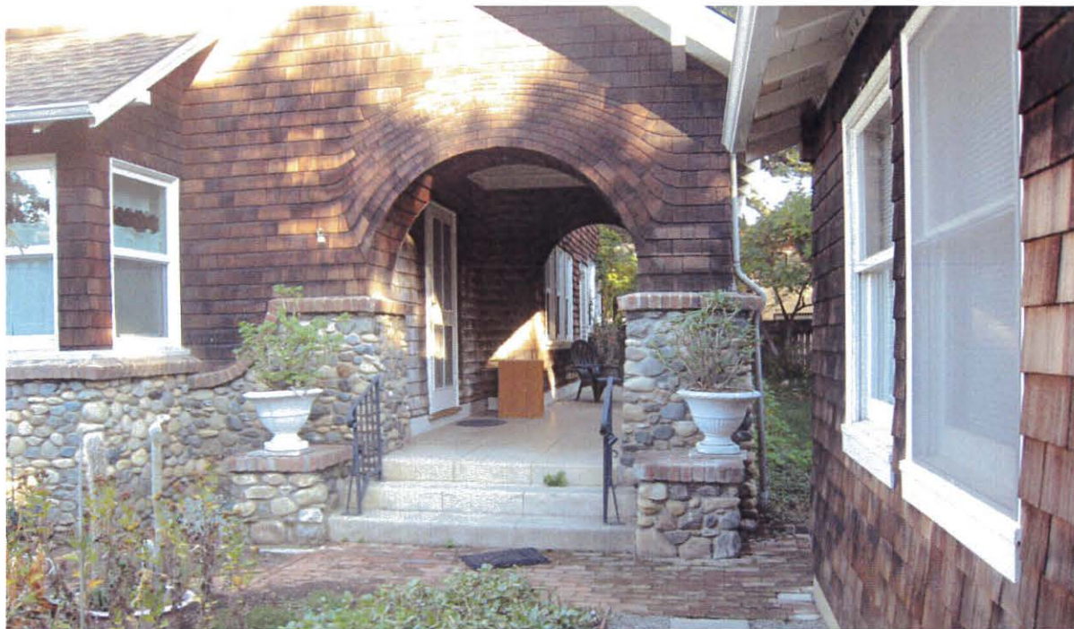
View of the house at the left and the garage/in-law unit at the right. Note the decorative shingles over the porch arch.
