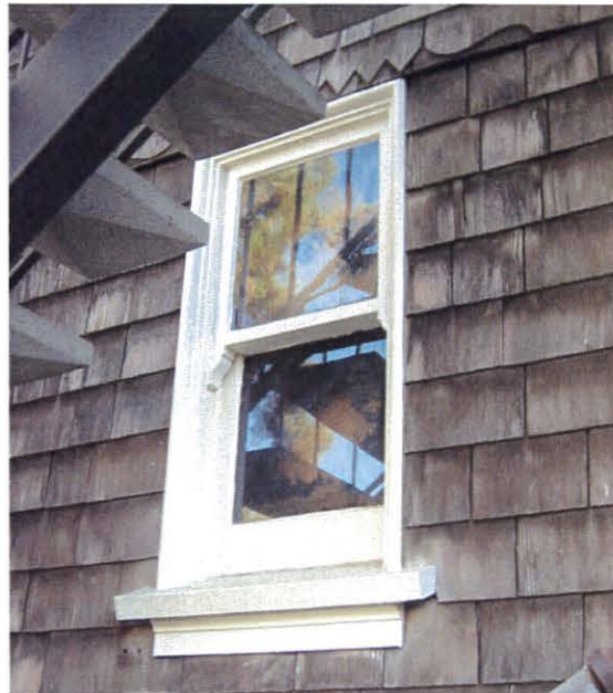
This is one of four windows proposed for removal from the first floor during phase 1. (The other three windows are at the north elevation: they are proposed to be replaced with doors.) This window illuminates the laundry room and is largely concealed behind the exterior staircase.
