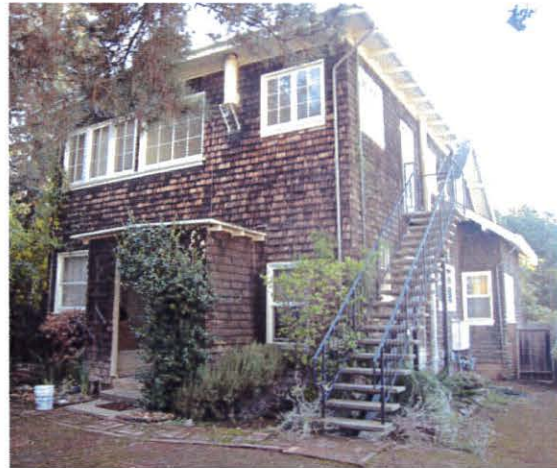
View of the west or rear elevation. Although this elevation is visible from Miravalle Avenue, the owner is proposing to replace all of the second floor windows with double-glazed, wood casement sash with interior and exterior grids to suggest the light configuration of the existing. The 12-light sash shown above is a fixed (inoperable) window; it is proposed for replacement with operable casement windows. The exterior staircase at the right will remain.
