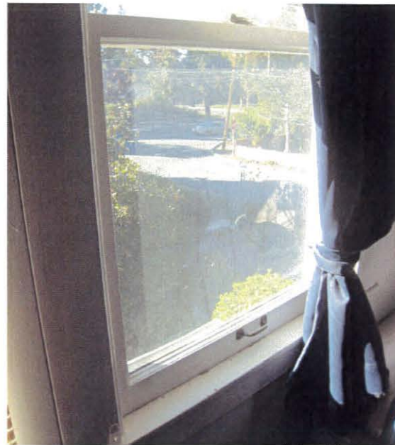
Interior view of the same windows.
