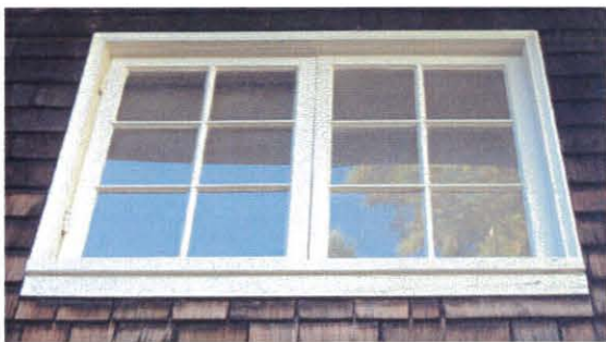
These are the westernmost casement sash in the south wall. They will be retained and possibly re-glazed with laminated glass with no tint.
