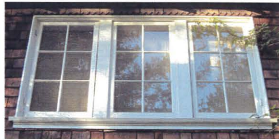
The above windows—the westernmost windows in this wall—will be replaced with double-glazed, wood casement sash with interior and exterior grids to suggest the same light configuration as the existing.
