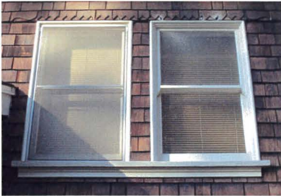
View of the existing second floor windows adjacent to the east porch. The windows will be replaced with double glazed wood four-over-four light sash with applied exterior and interior grids to suggest four lights per sash. Please see window cut sheets incorporated into the drawings for section details.
