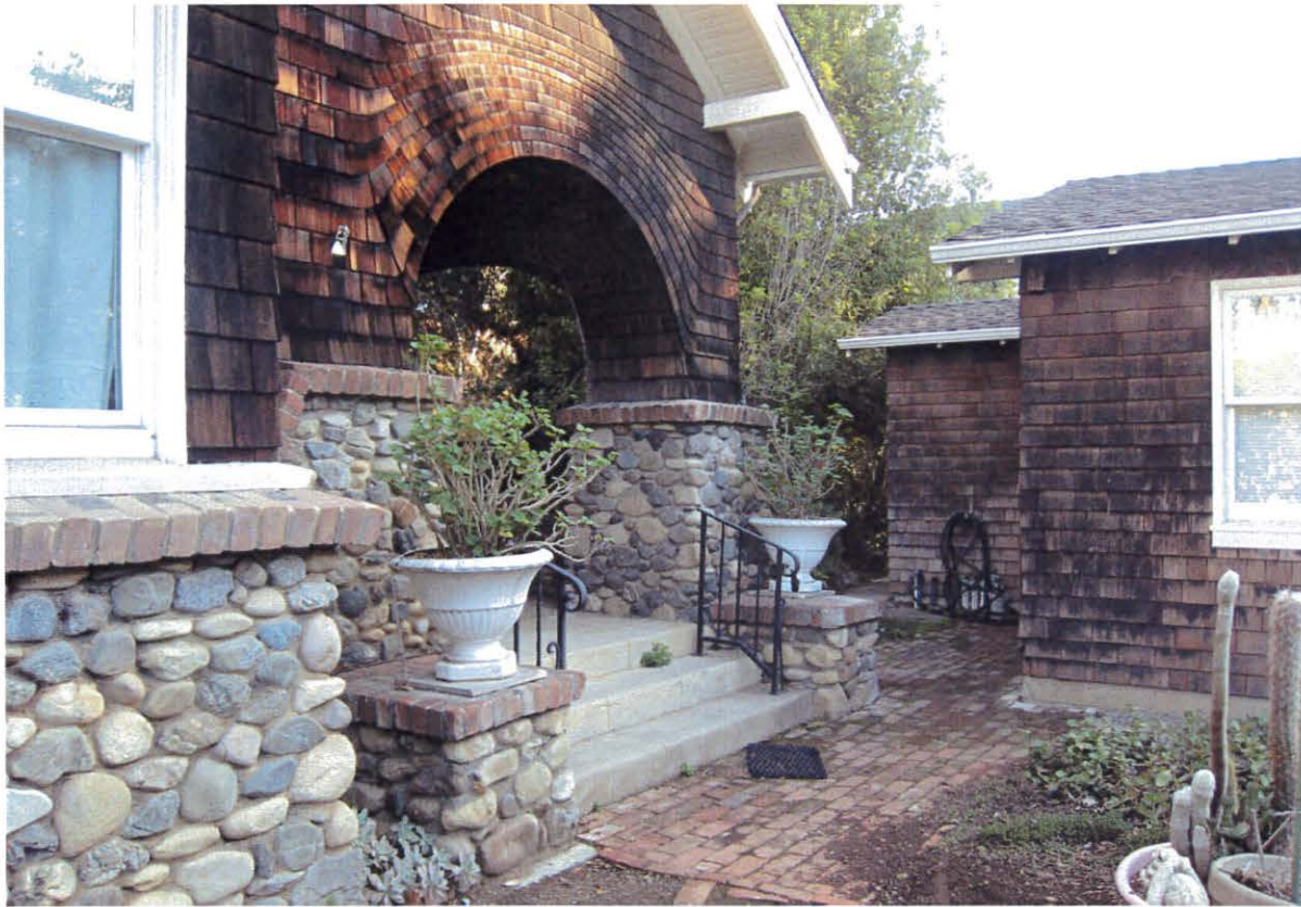
View of the house at the left and the garage/in-law unit at the right.
