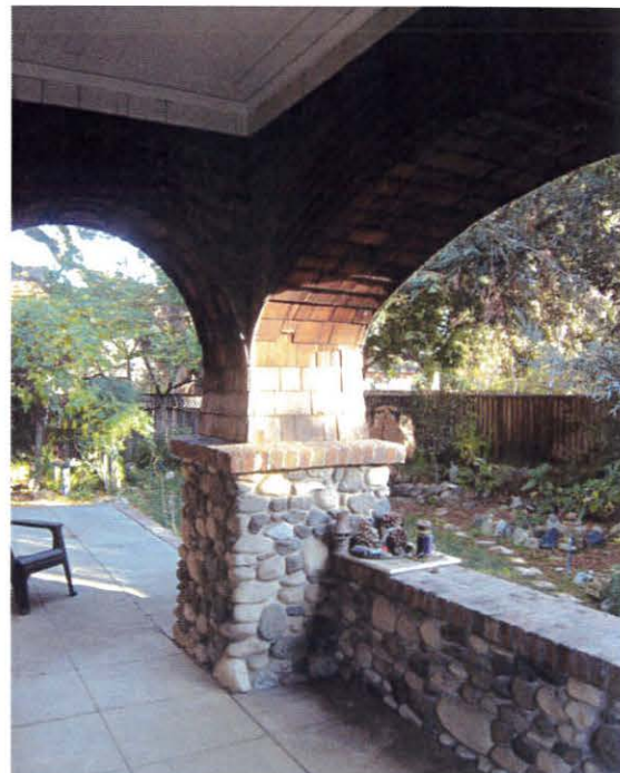
View from the porch into the side garden.
