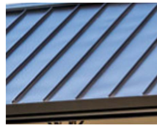
SHEET METAL ROOFING
