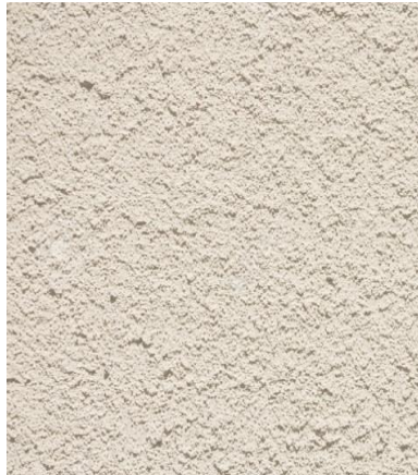
STUCCO WALL FINISH PAINTED WITH KM5759 COLOR
