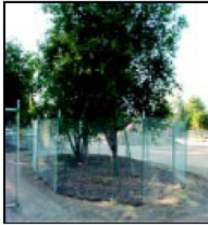
IMAGE 2.15-1 Tree Protection Fence at the Dripline
