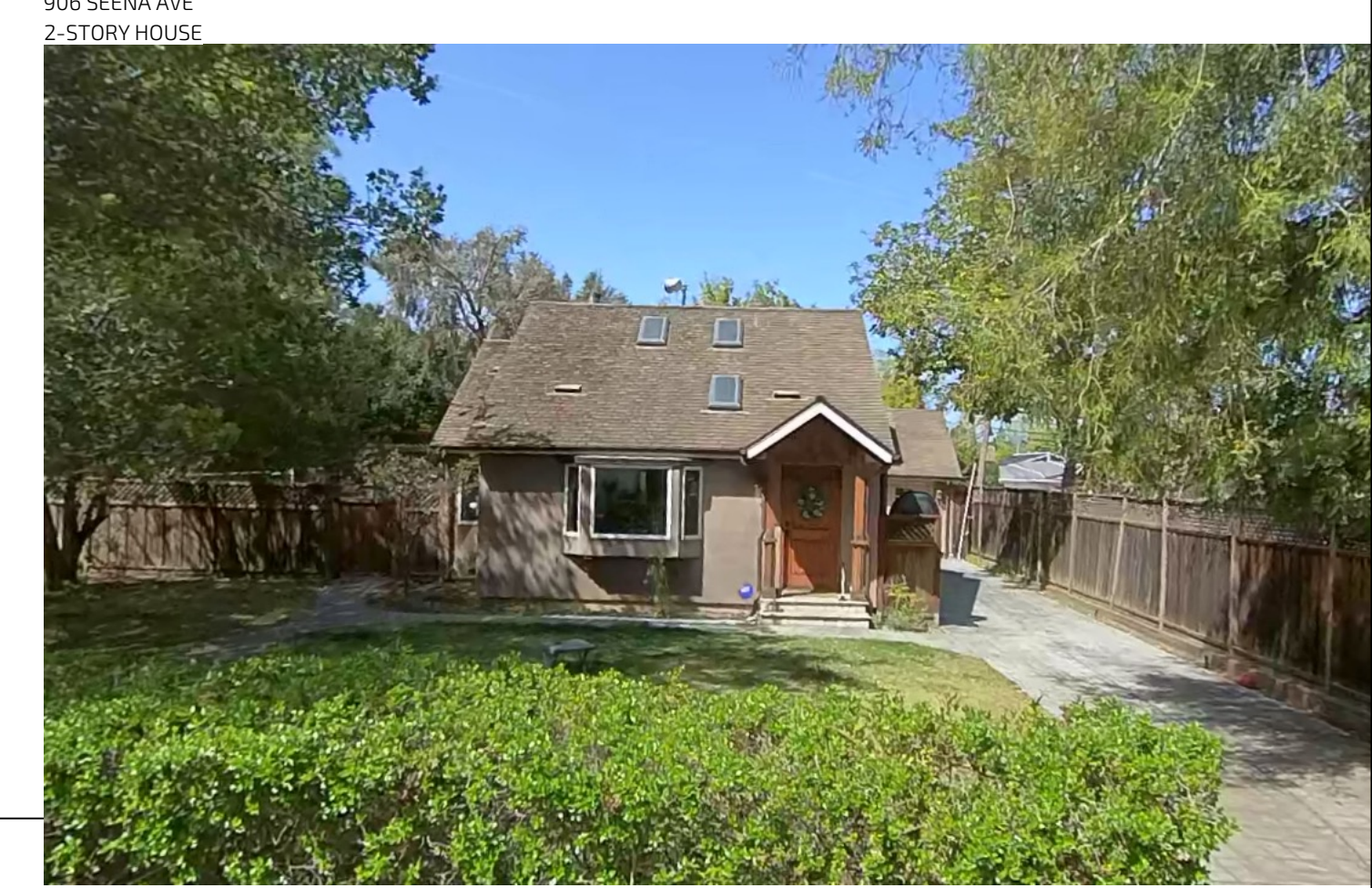
906 SEENA AVE 2-STORY HOUSE
