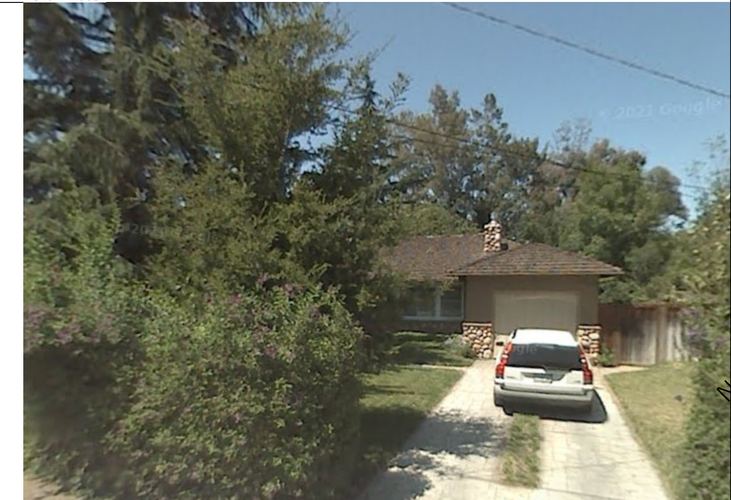
916 SEENA AVE 1-STORY HOUSE
