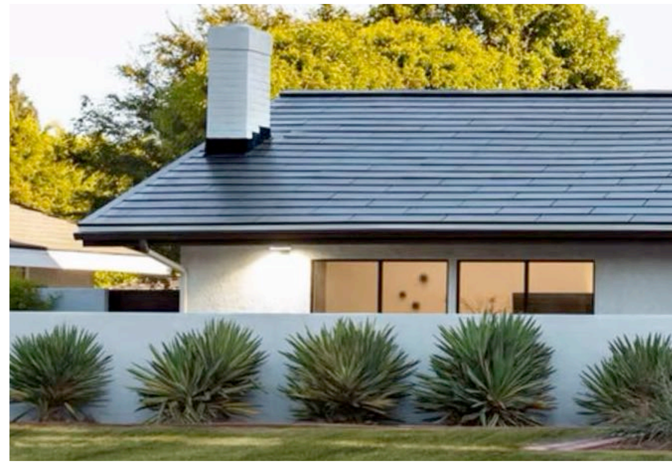
ROOF @ Second Floor TESLA Solar Roof System
