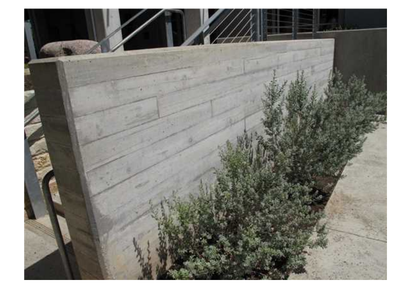
Concrete Wall (In Front ADU) (Reference Image)
