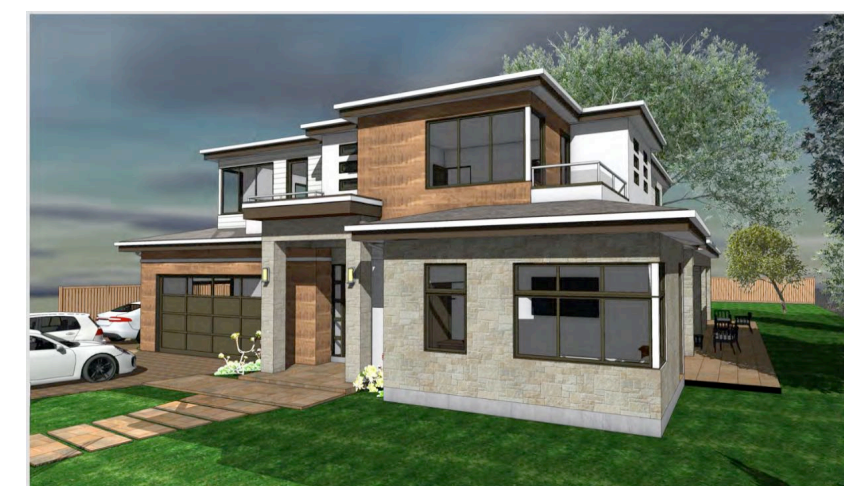
960 PARMA WAY (UNDER CONSTRUCTION)
