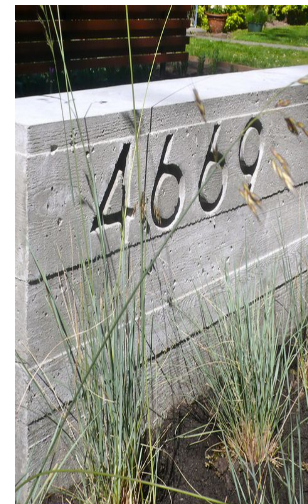
EXTERIOR LOW WALLS @ ADU 4' Height Board-formed Concrete Low Wall @ Covington Rd in front of ADU
