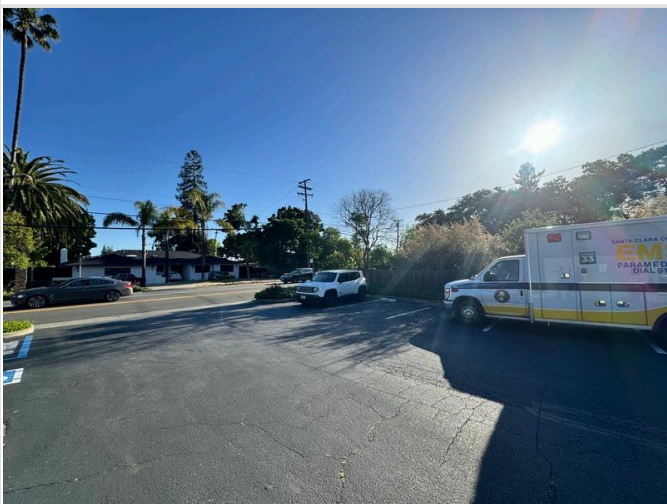
59. Cracks and alligating observed on the pavement
