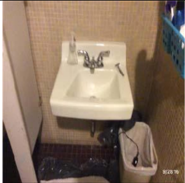
D2013 Lavatories:- View of Wall Hung Lavatories
