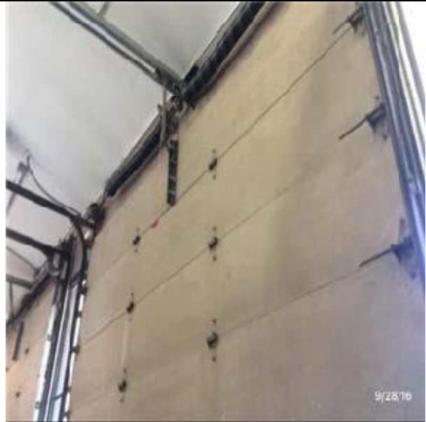
B2034 Overhead Doors:- View of Rolling Overhead Doors, Electric
