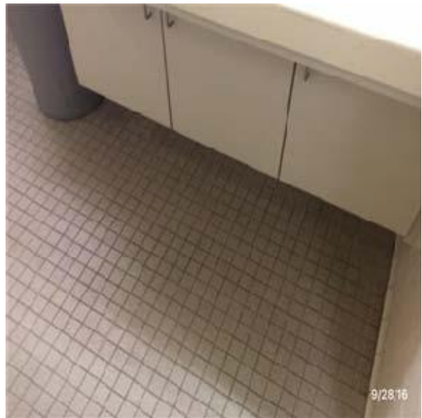
C3024 Flooring:- View of Ceramic Tile
