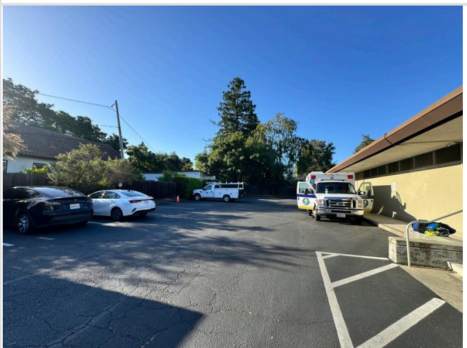
60. Cracks and alligating observed on the pavement
