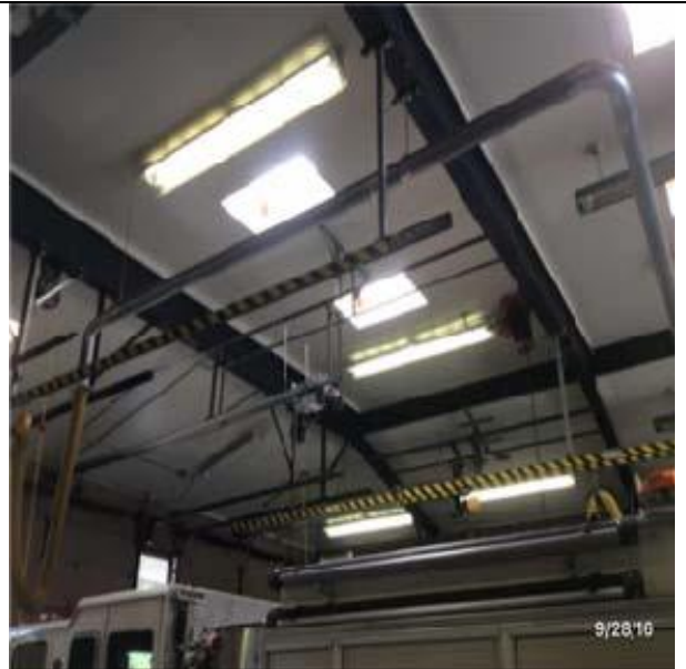
B1022 Pitched Roof Construction:- View of Steel Beams and Rafters
