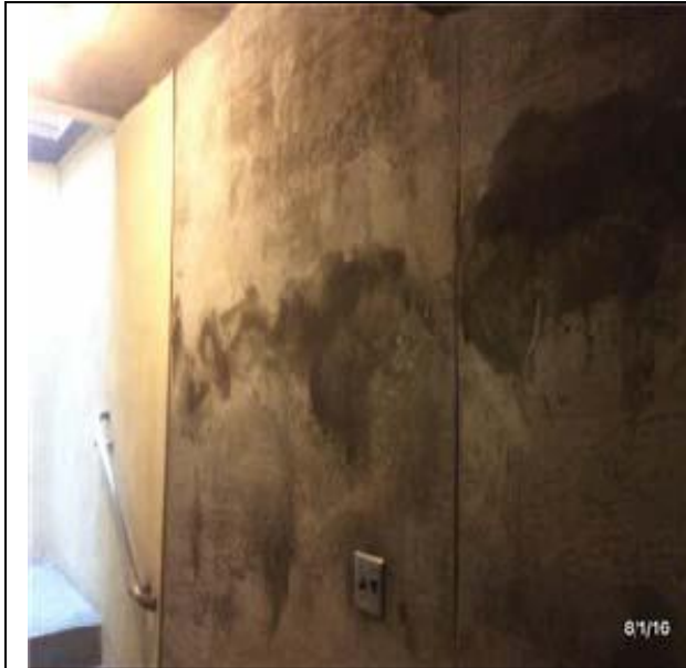
A2021 Basement Wall Construction:- View of Basement Construction
