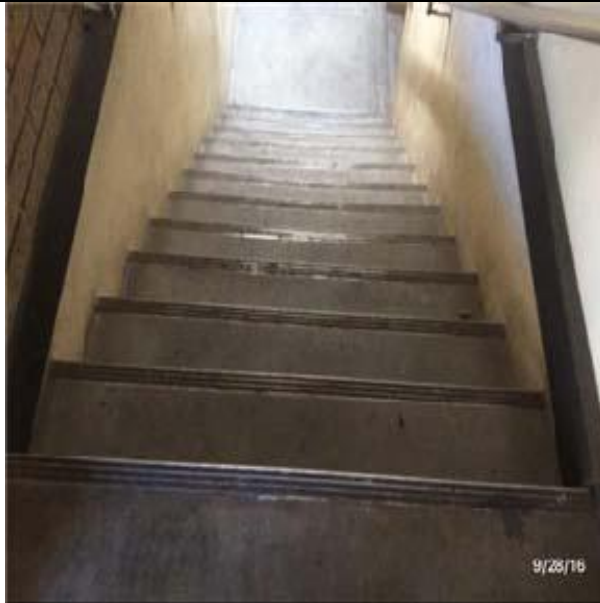
C2011 Regular Stairs:- View of Regular Stairs – Concrete Construction
