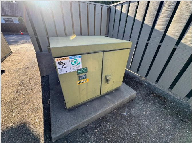
52. Pad-mounted transformer
