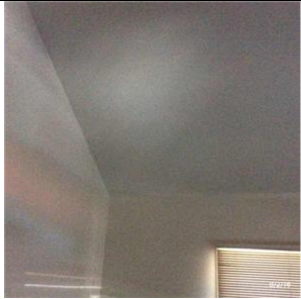
C3031 Ceiling Finishes:- View of Gypsum Wall Board Ceilings
