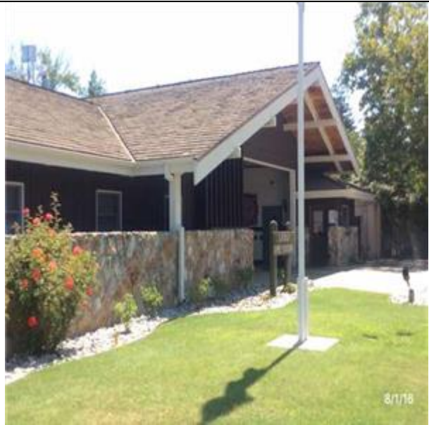
B2011 Exterior Wall Construction:- View of Veneer – Stone
