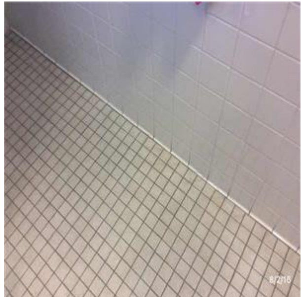
C3024 Flooring:- View of Ceramic Tile
